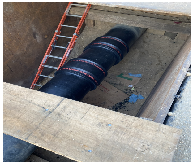
Replaced Pipe Joint on Emma St
