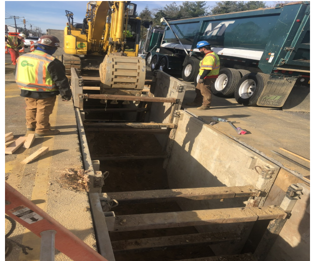
Excavating and Installing Trench Boxes on Central Ave
