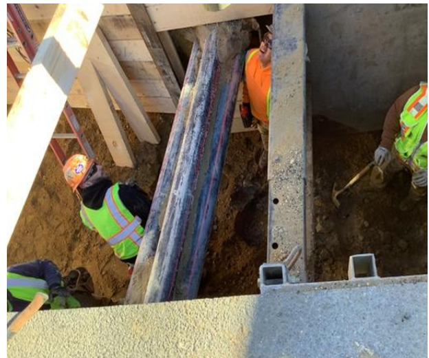
Excavating Pipe Trench under Conduits on Central Ave
