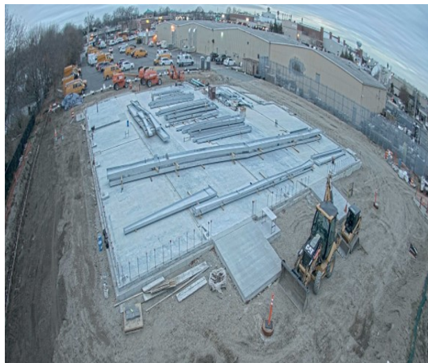
Aerial View from East Side of Site
