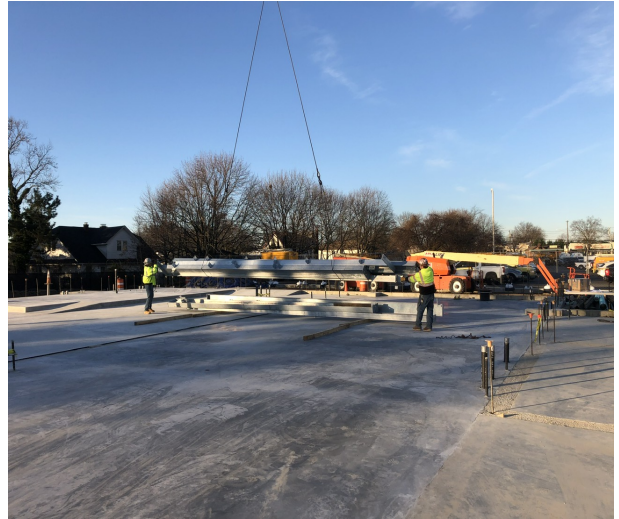
Staging Building Steel Components
