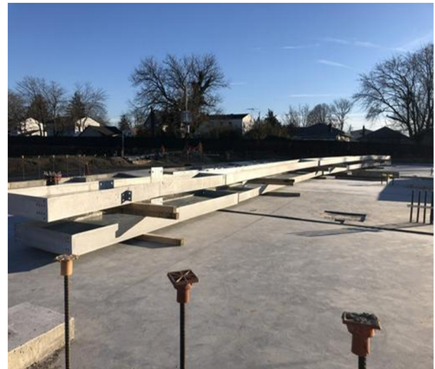
Assembled Building Roof Truss Staged for Installation
