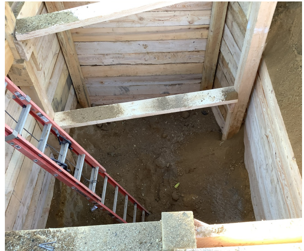
HDPE Pipe Fusion Pit on Central Ave
