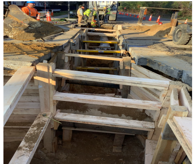
Shoring and Trenching on Central Ave
