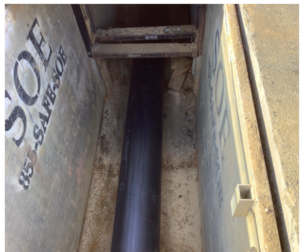
Installed HDPE Pipe on Central Ave
