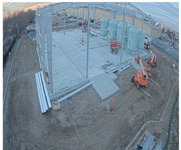
Aerial View from East Side of Site
