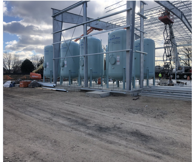
Carbon Units Installed on Building Floor Slab
