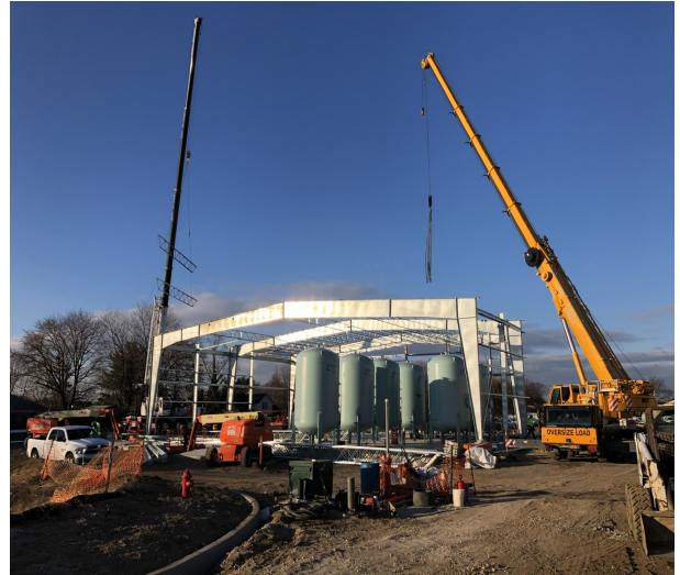
Installing Building Structural Steel
