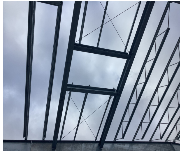
Building Roof Framing for Ventilation Fan
