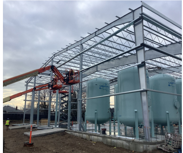
Installing Building Structural Steel
