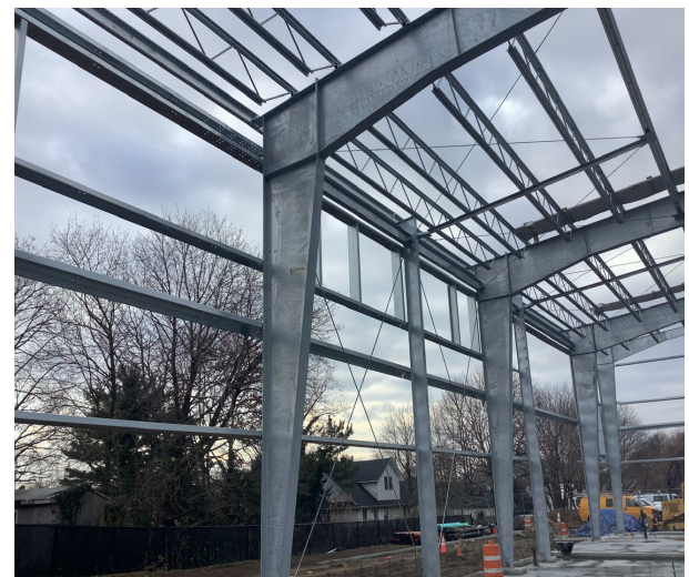
Framing for Building Windows
