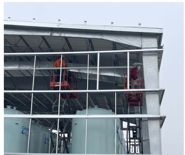
Installing HVAC Duct Above Carbon Units
