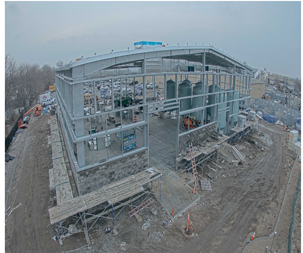
Aerial View from East Side of Site
