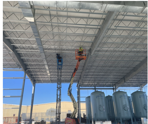
Installing Sprinkler System Piping
