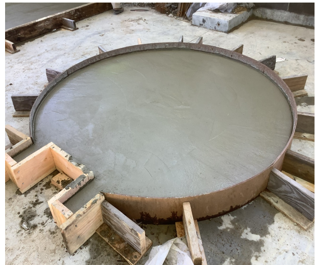
Concrete Equipment Pad
