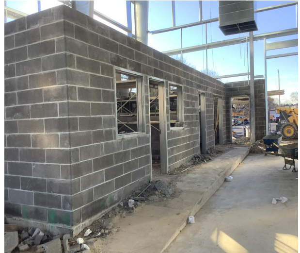
Block Walls for Office Area
