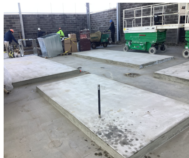
Completed Concrete Equipment Pads
