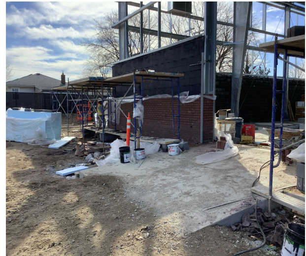
Installing Brick on East Exterior Wall
