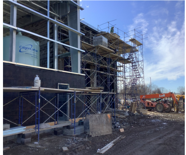
North Exterior Wall
