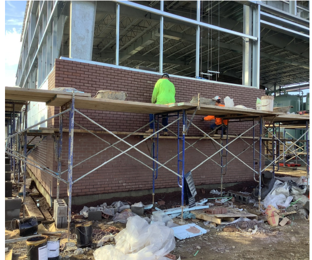
Installing Brick on East Exterior Wall
