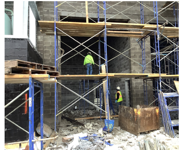
Completing Chemical Room Block Walls
