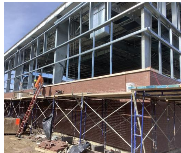
Installing Brick Precast Concrete Caps on South Wall
