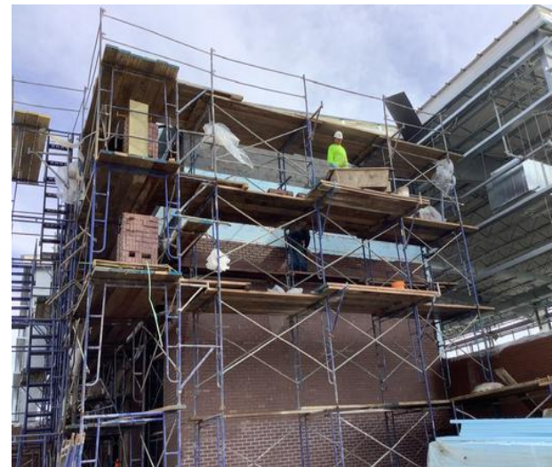
Installing Bricks on Chemical Room Exterior Wall
