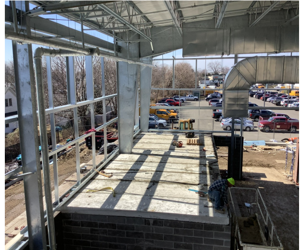
Installing Precast Concrete Roof Planks on Interior Rooms
