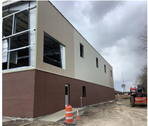
Completed Brick and Metal Wall Panels on South Side
