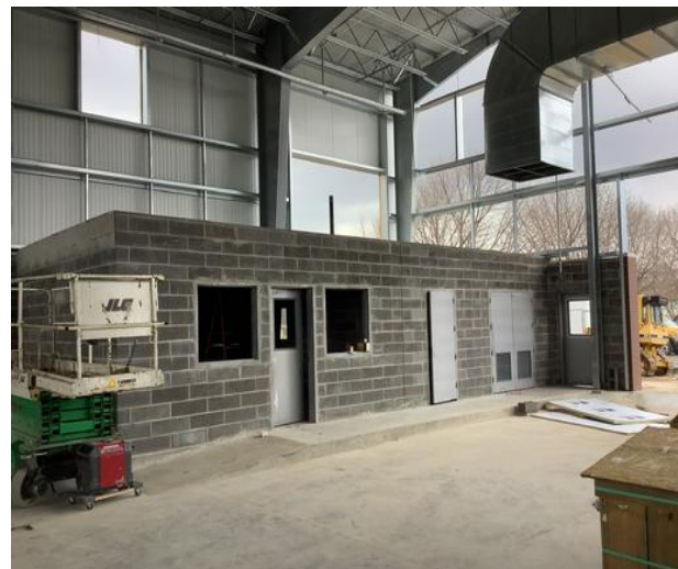
Interior Rooms with Doors Installed
