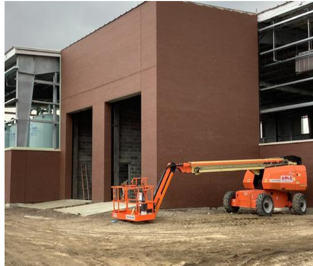
Completed Brick Walls at Chemical Rooms
