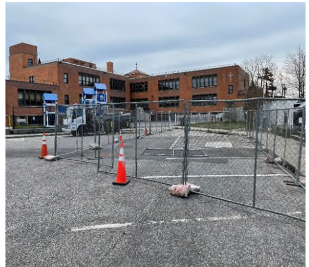
RW-21 Staging Area Setup
