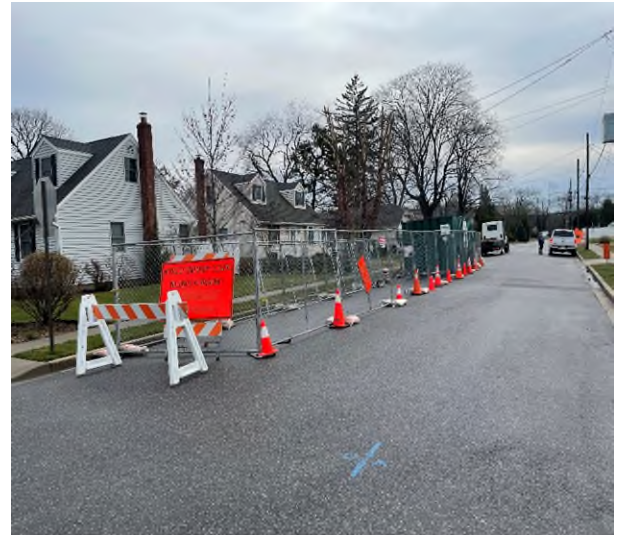
RW-20 Staging Area with 10,000-Gallon Frac Tank On-site
