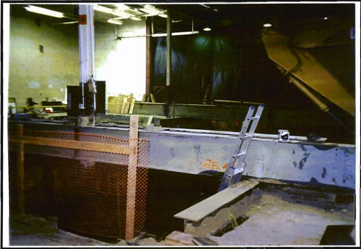
Photo 7: Building Column Needle Beam supports above excavation pit.
