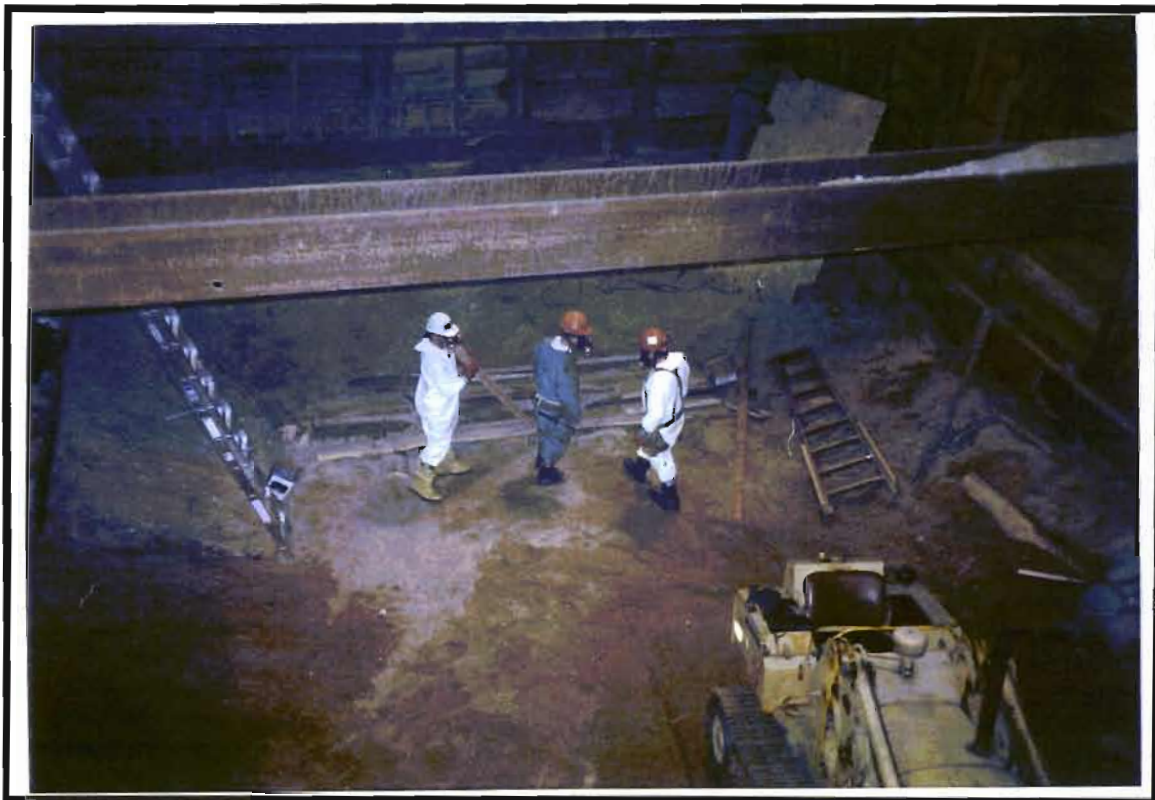
Photo 12: Timber lagging being measured and cut prior to installation.
