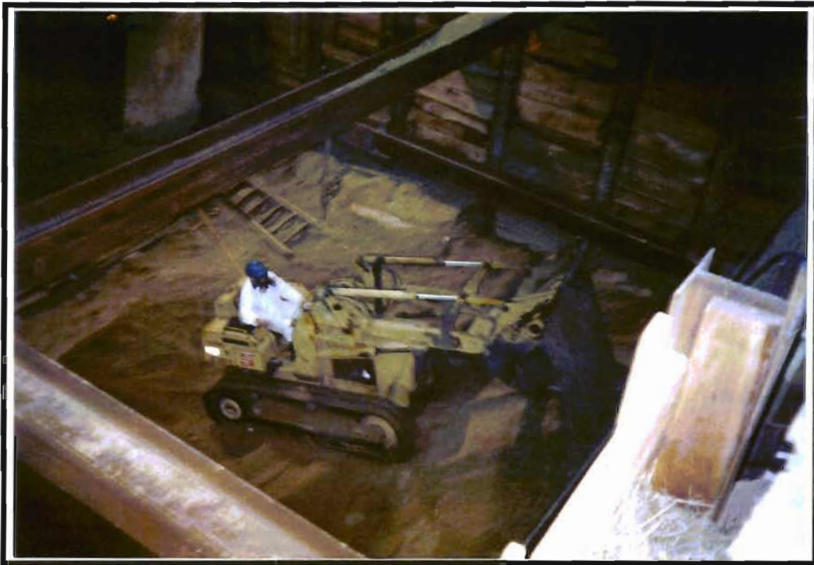
Photo 11: Tracked dozer in pit excavating.
