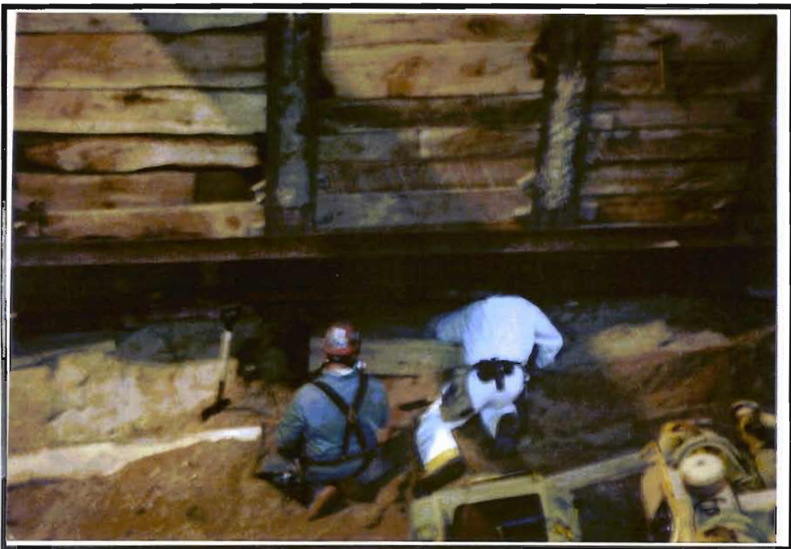
Photo 6: Installation of Timber Lagging.
