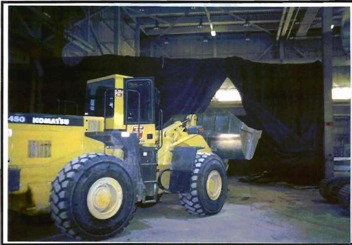
Photo 13: Front-End Loader stockpiling excavated soil.
