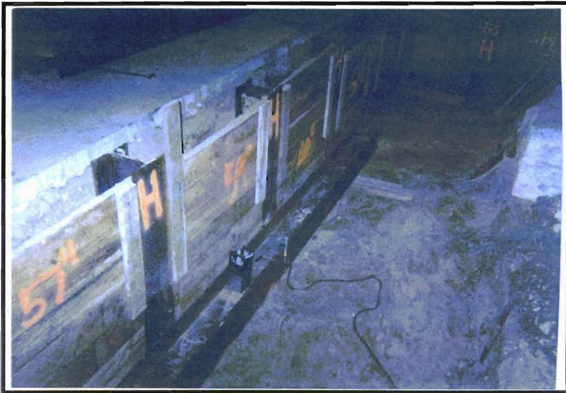
Photo 5: Steel Whaler and timber lagging in place.
