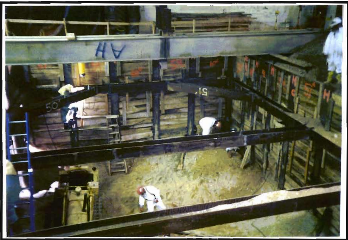
Photo 10: Welding, excavating, and timber lagging.
