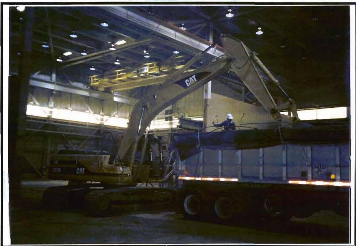
Photo 14: Hydraulic Excavator loading excavated soil into truck for disposal.
