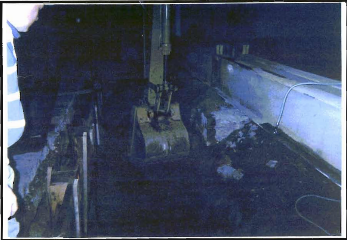
Photo 3: Excavation around Building Column Footer.
