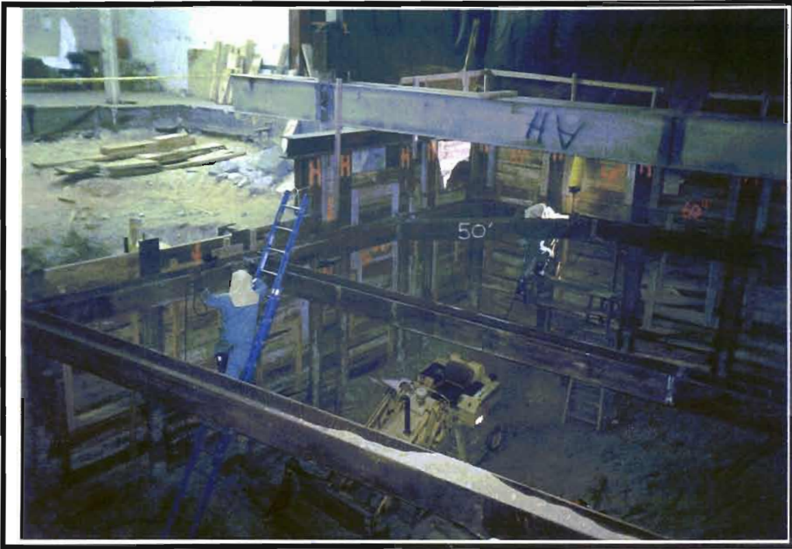
Photo 9: Welding of Cross Bracing to Whalers.
