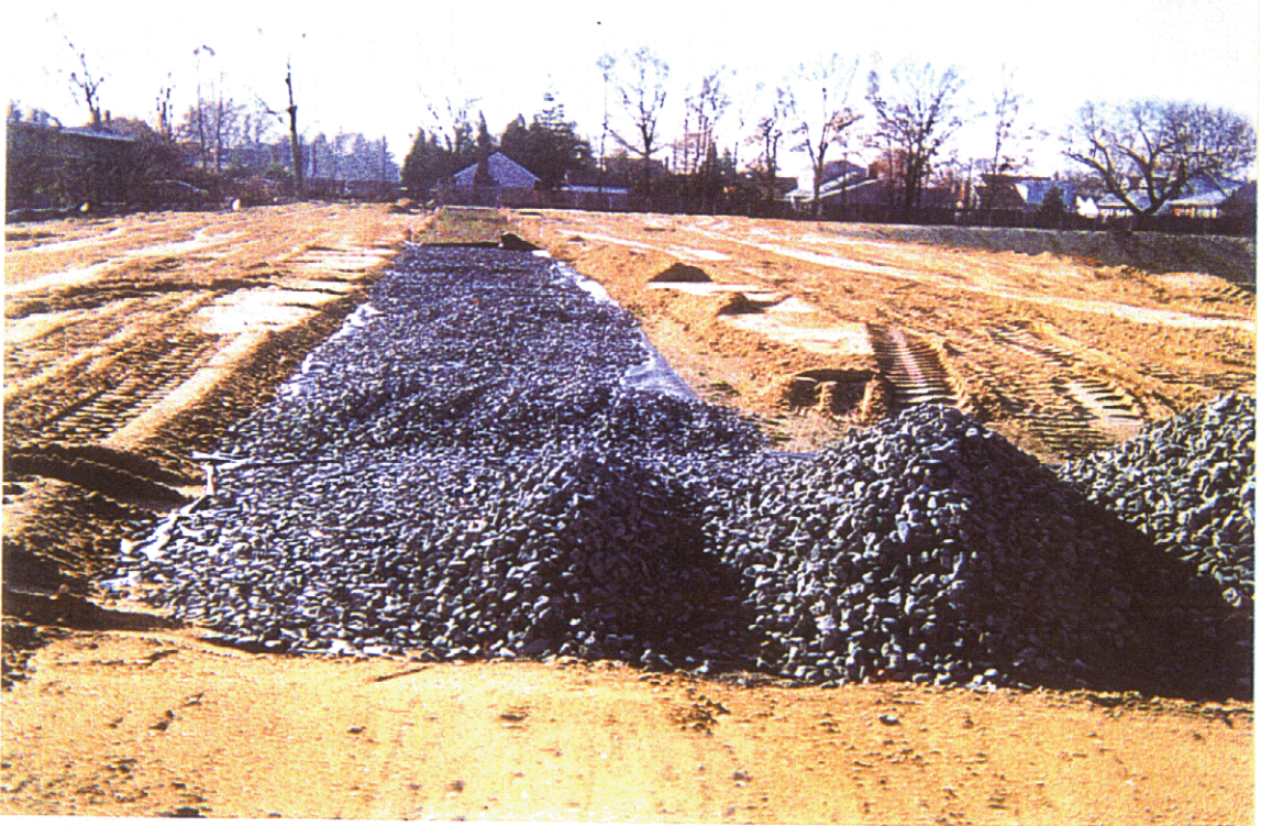
EASTERN ACCESS ROAD CONSTRUCTION, LOOKING SOUTH. SOIL COVER MOSTLY COMPLETE ON SIDES
