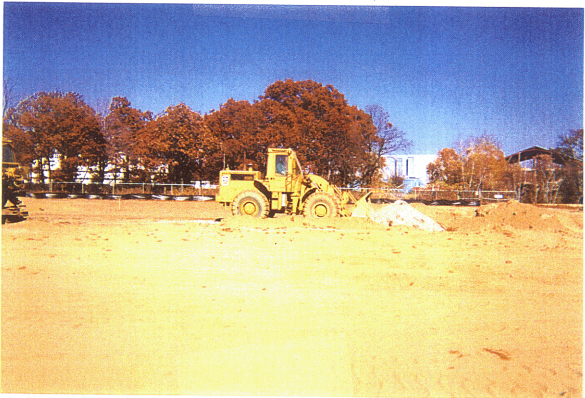
SOIL COVER, LOOKING NORTH TOWARD FORMER SLUDGE DRYING BEDS (PRE RAIN)
