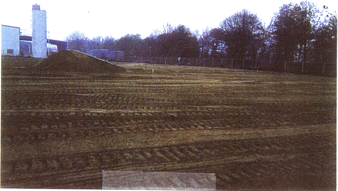
SOIL COVER, LOOKING WEST TOWARD FORMER SLUDGE DRYING BEDS
