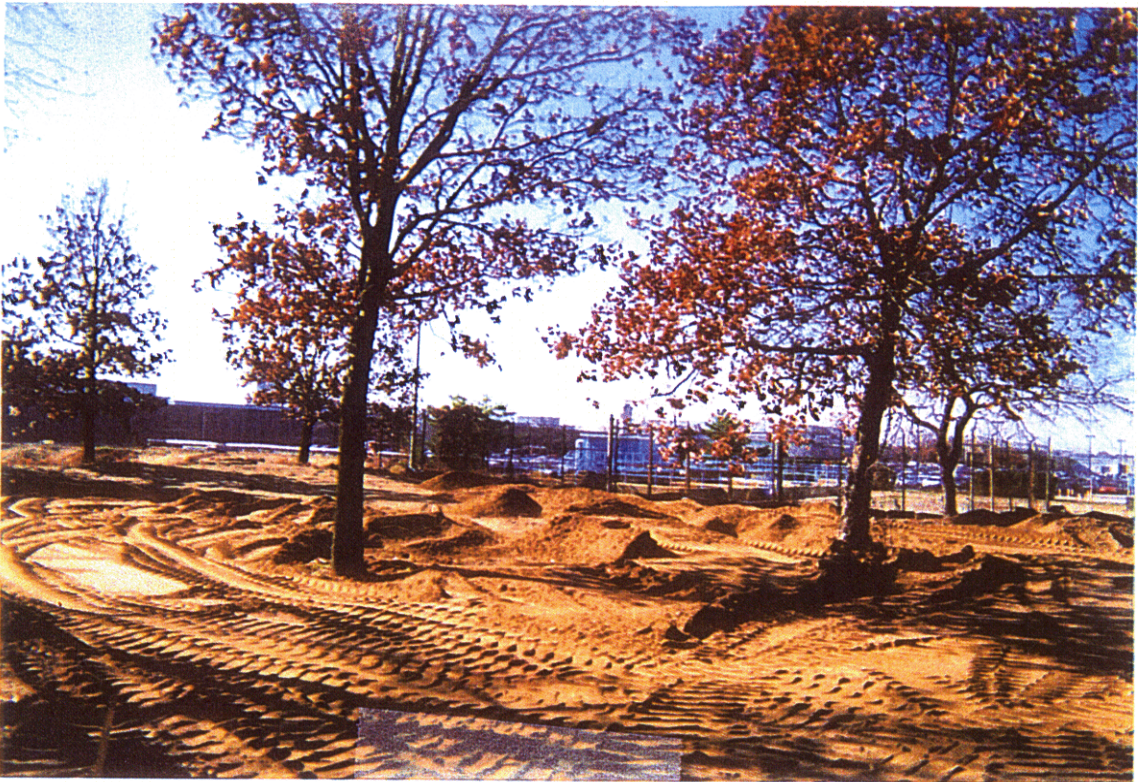
SOIL COVER EAST OF SALT SHED, LOOKING SOUTHWEST TO PLANT NO. 3
