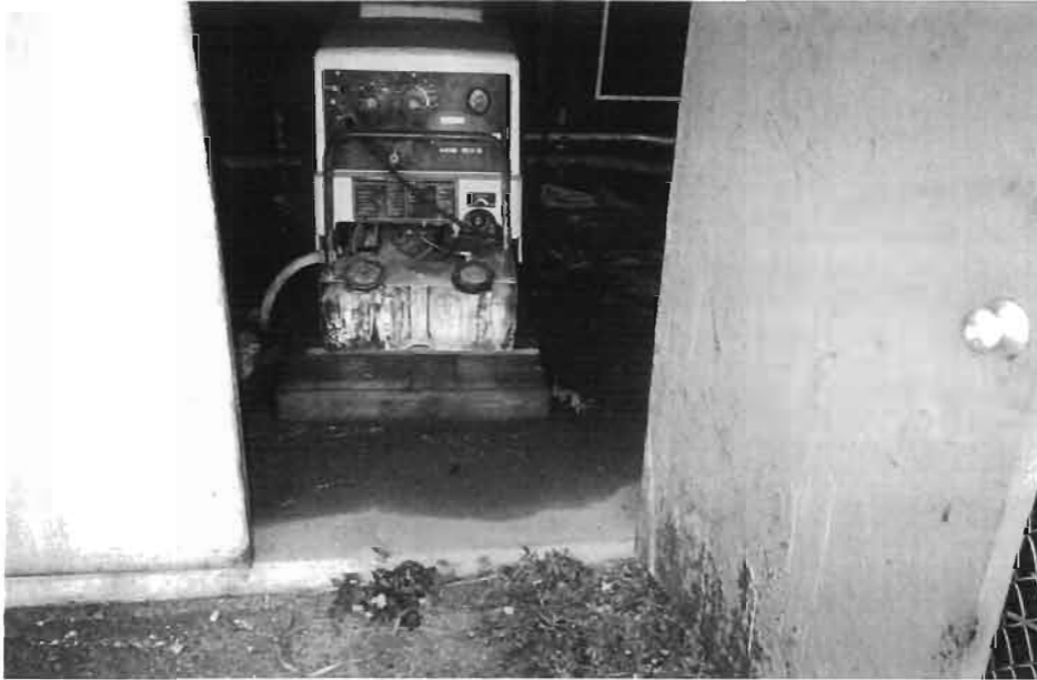
Photo 7: Steam Jenny in Building 20-03
