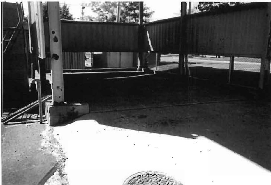
Photo 6: Exterior Vehicle Wash Rack (Building 20-04)
