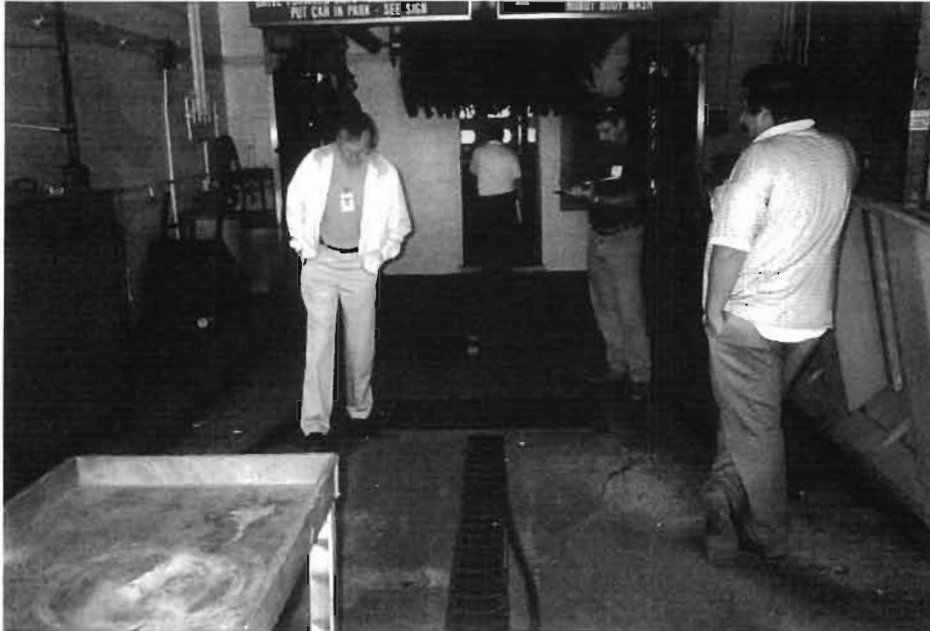
Photo 5: Interior Vehicle Wash Bay in Building 20-01
