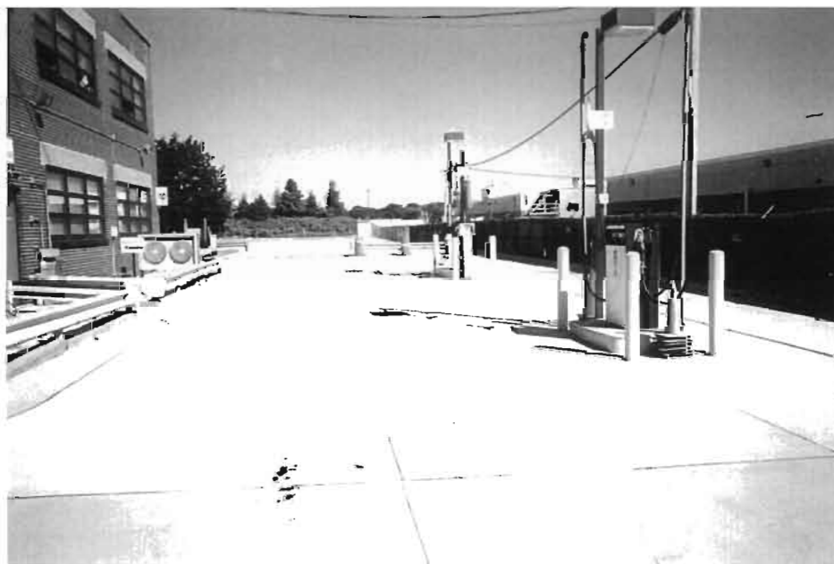
Photo 2: Fuel Pumps on South Side of Building 20-01
