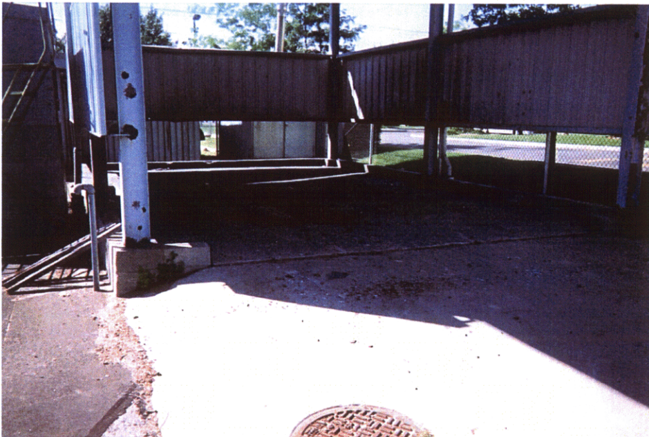
Photo 6: Exterior Vehicle Wash Rack (Building 20-04)
