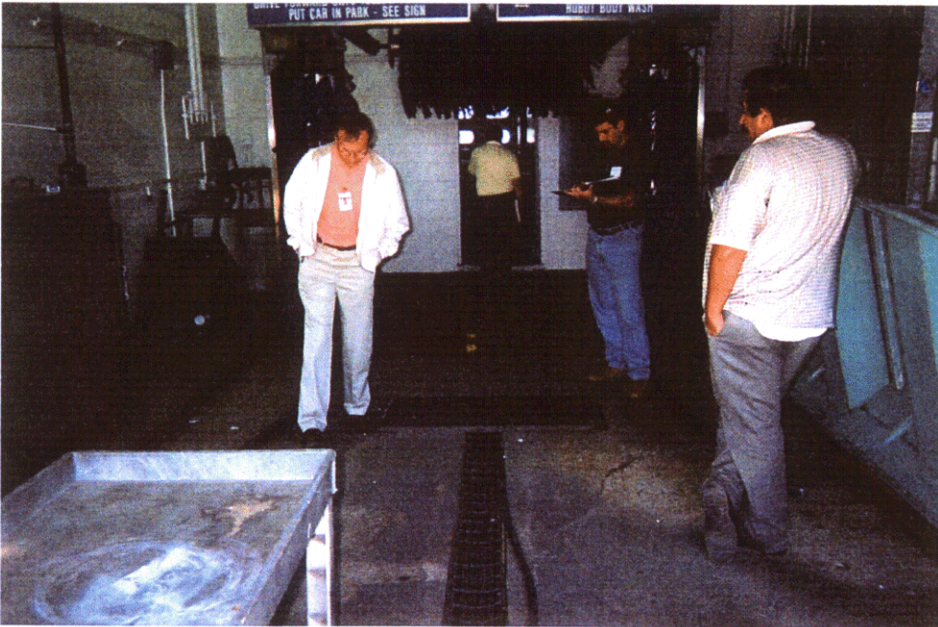
Photo 5: Interior Vehicle Wash Bay in Building 20-01
