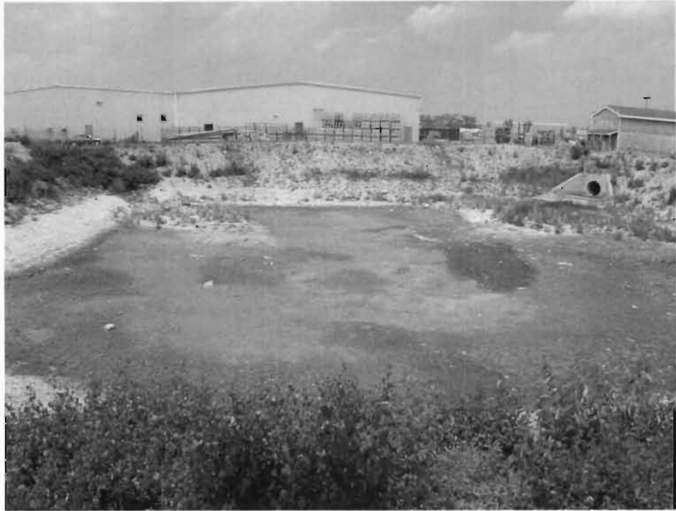
South Receiving Basin Looking North.
