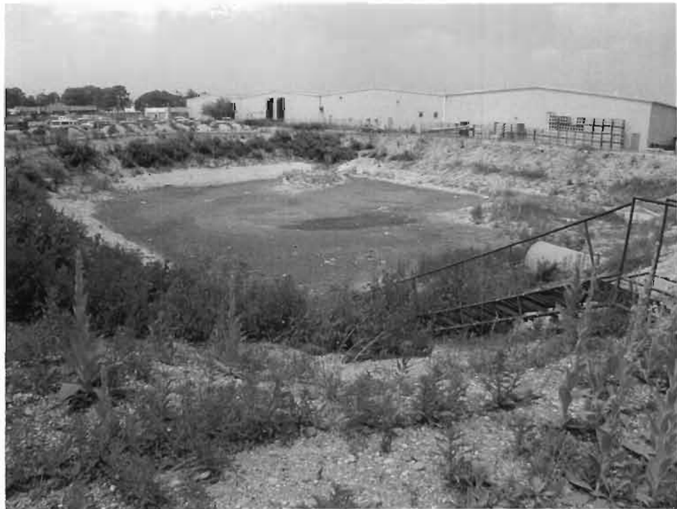
South Receiving Basin Looking Northwest.
