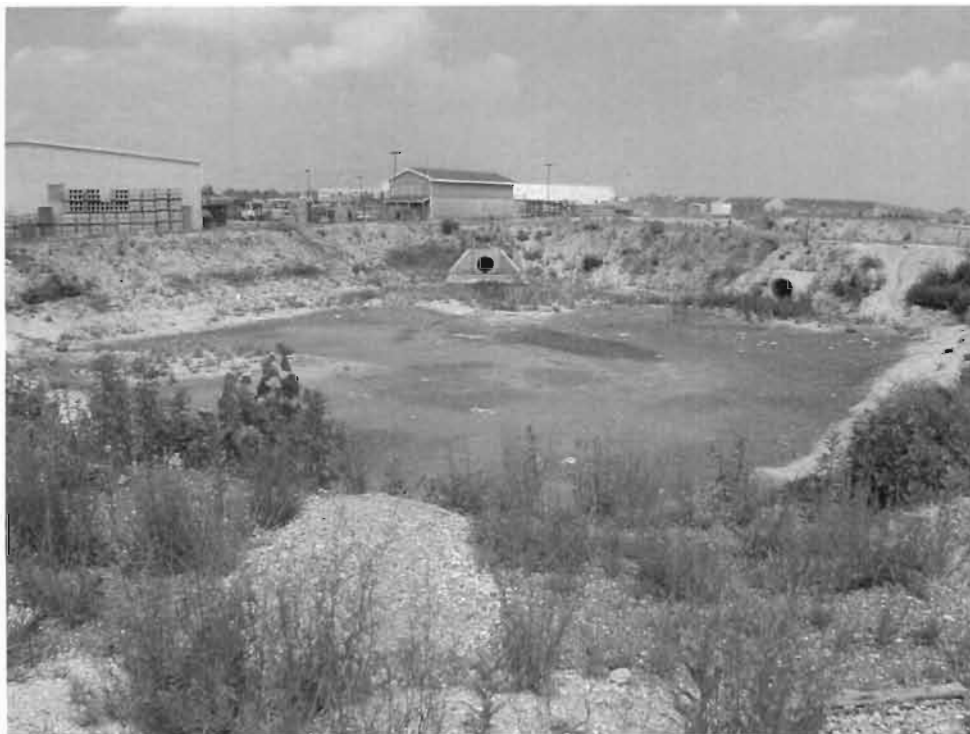
South Receiving Basin Looking Northeast.
