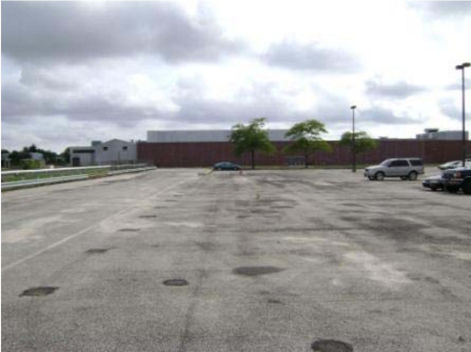
Photo 11 – Site 3, western portion of Impound Lot 1, looking south.
