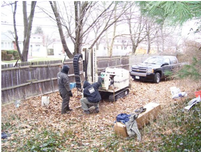
Photo 2: DPT rig, East of Site 1
