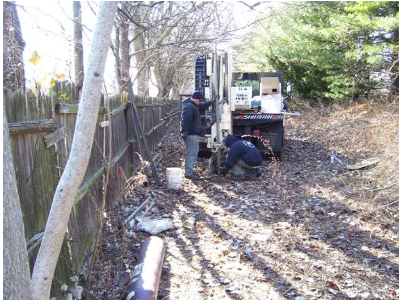
Photo 5: DPT rig, East of Site 1
