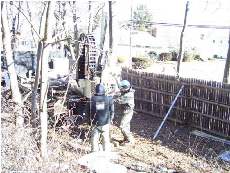
Photo 1: DPT rig, East of Site 1
