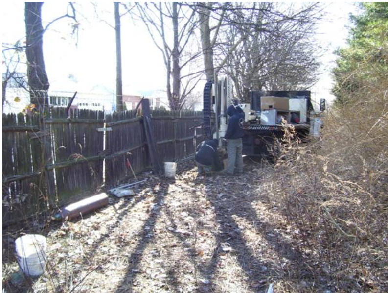
Photo 6: DPT rig, East of Site 1
