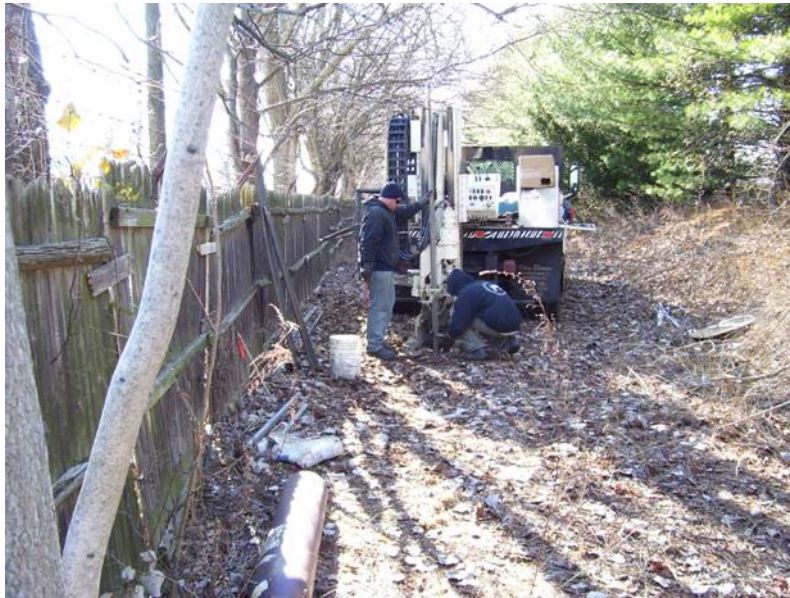
Photo 5: DPT rig, East of Site 1
