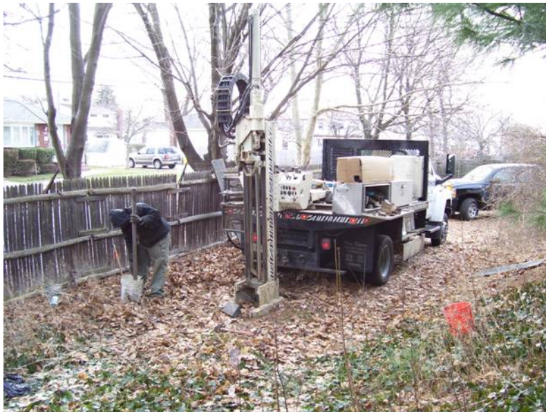
Photo 4: DPT rig, East of Site 1
