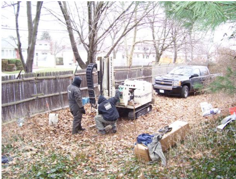
Photo 2: DPT rig, East of Site 1
