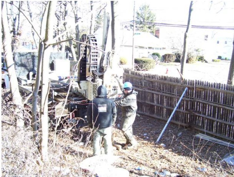
Photo 1: DPT rig, East of Site 1
