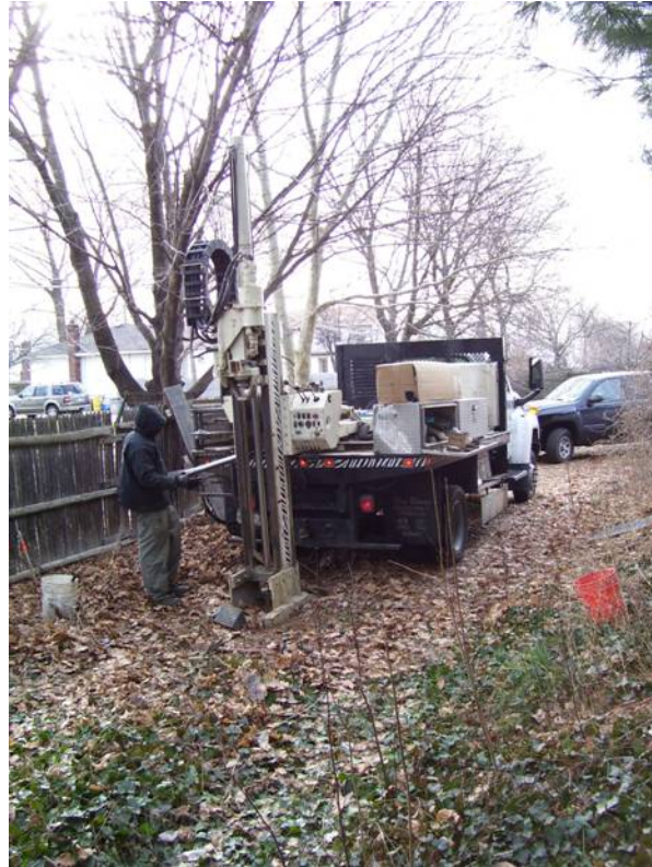
Photo 3: DPT rig, East of Site 1
