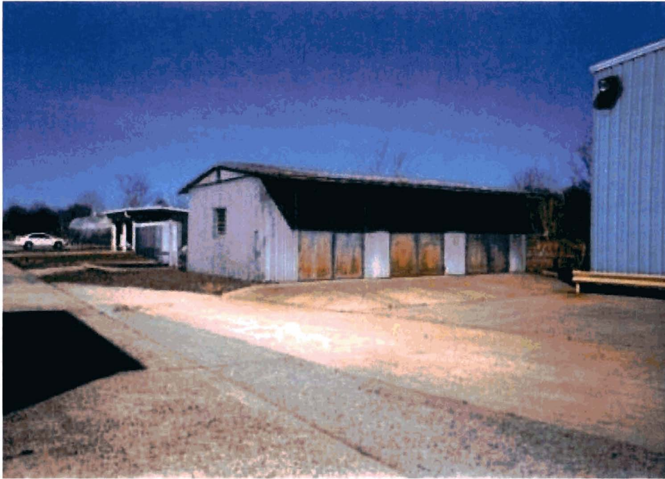
Photo 1 – Site 1, metal buildings, southwest concrete pad situated in the southwestern portion of the Site, looking northeast.
