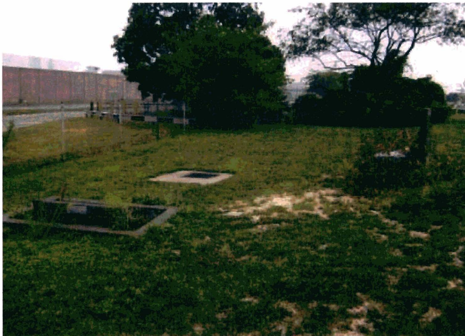
Photo 10 – Site 2, storm water diverter situated in the southeast portion of the Site.
