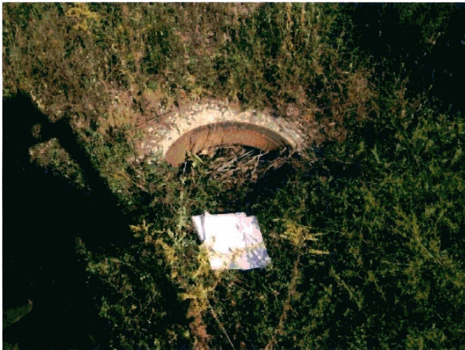
Photo 6 – Site 1, former cesspool.
