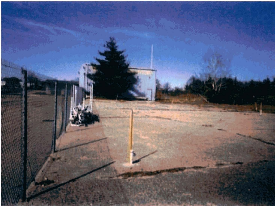
Photo 2 – Site 1, southwest concrete pad situated in the southwestern portion of the site, looking north
