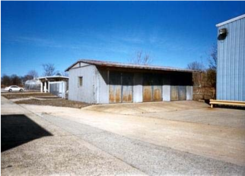
Photo 1 – Site 1, metal buildings, southwest concrete pad situated in the southwestern portion of the Site, looking northeast.
