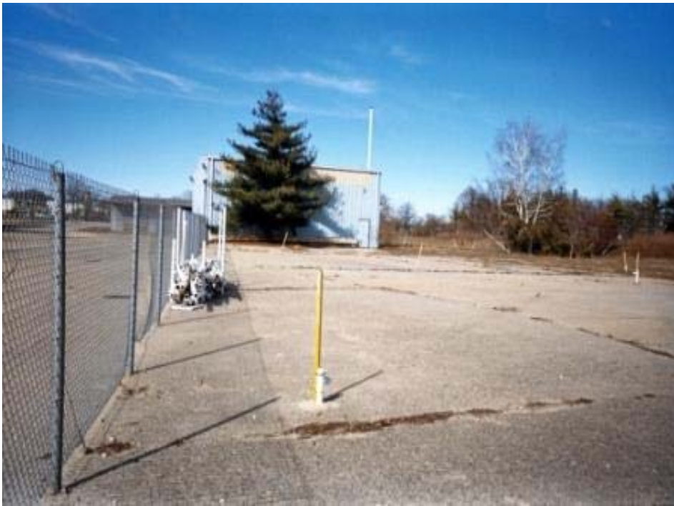
Photo 2 – Site 1, southwest concrete pad situated in the southwestern portion of the site, looking north
