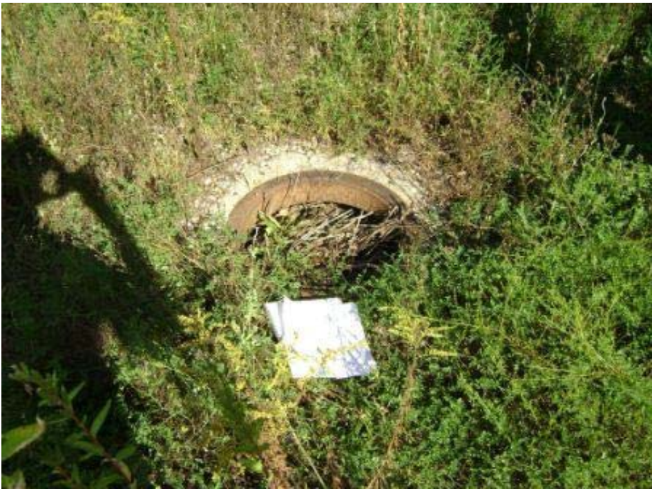
Photo 6 –Site 1, former cesspool.
