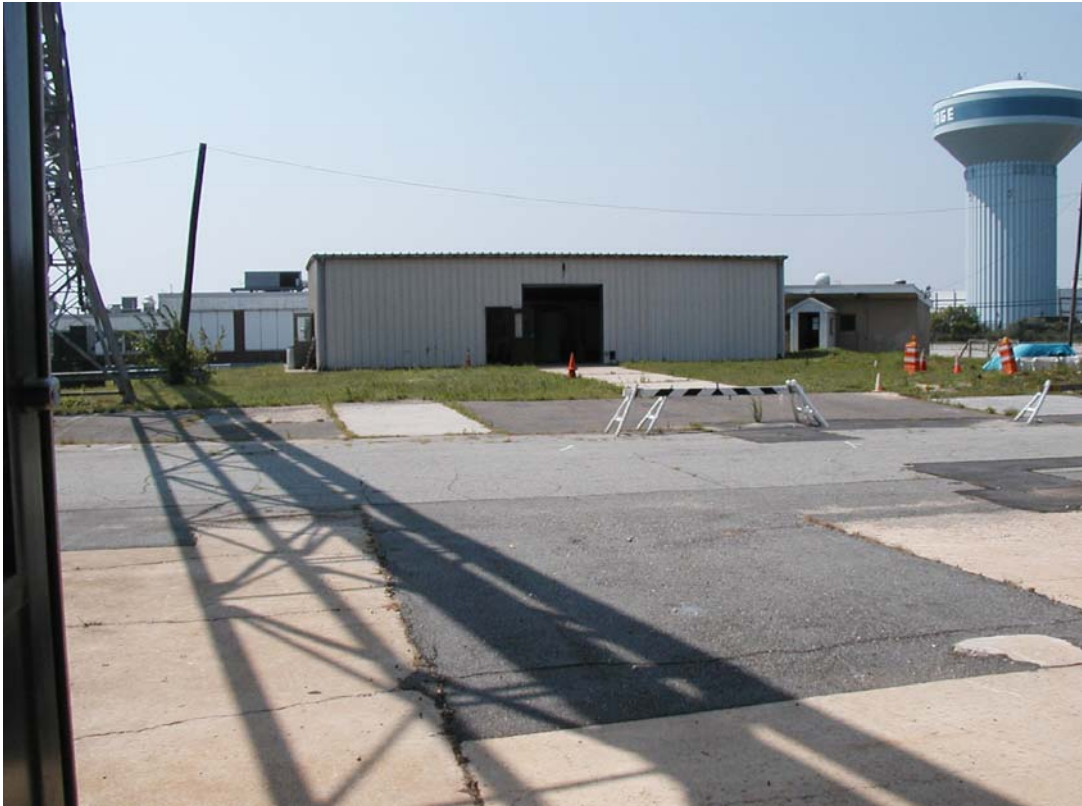
Site 4 -Proposed Treatment Building, looking south
