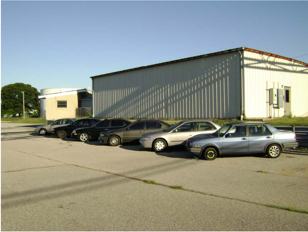
Site 4 – Proposed Treatment Building, looking northwest
