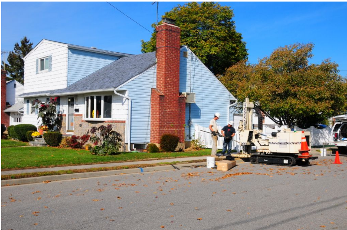
Photo 4: Looking – at DPT rig positioned at BPS1-SG2005
