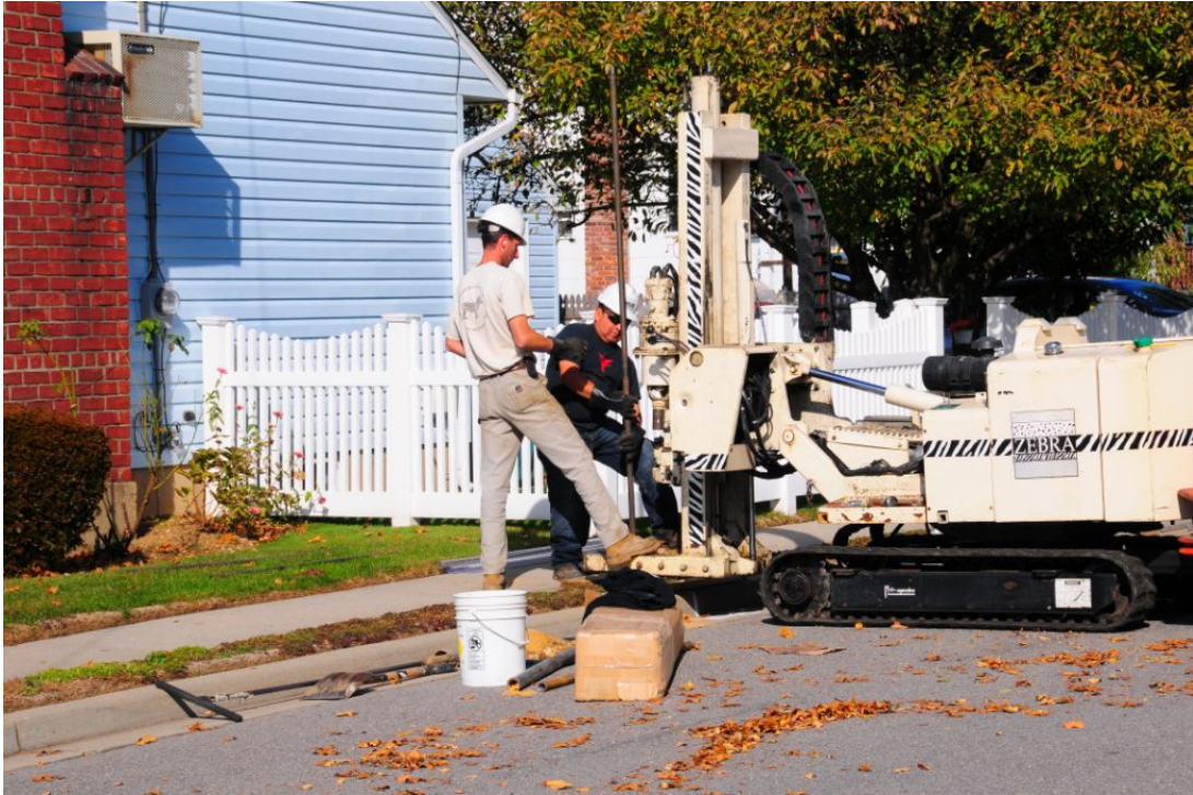
Photo 3: Close up view of DPT rig at BPS1-SG2005.
