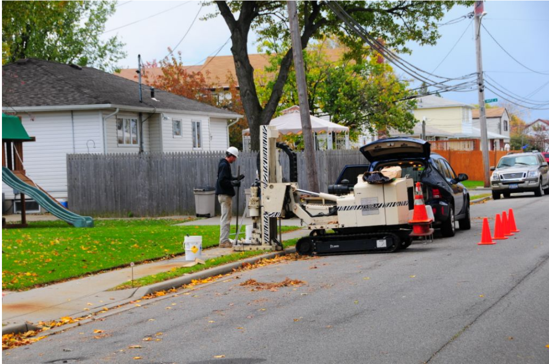
Photo 7: Looking SE at DPT rig positioned at BPSI-SG2002.
