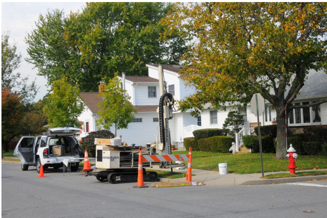
Photo 1: DPT rig, East of Site 1 positioned at BPSI-SG2008.
