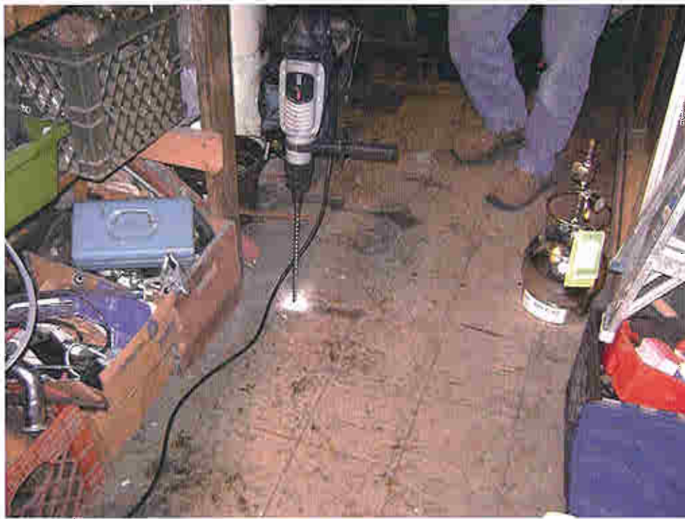
Photo 32: Drilling of basement floor to collect sub-slab sample at Home #9.
