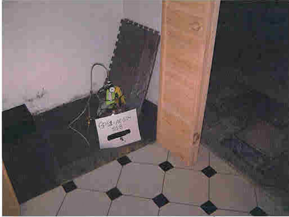
Photo 49: Sub-slab sample location in Home #14.
