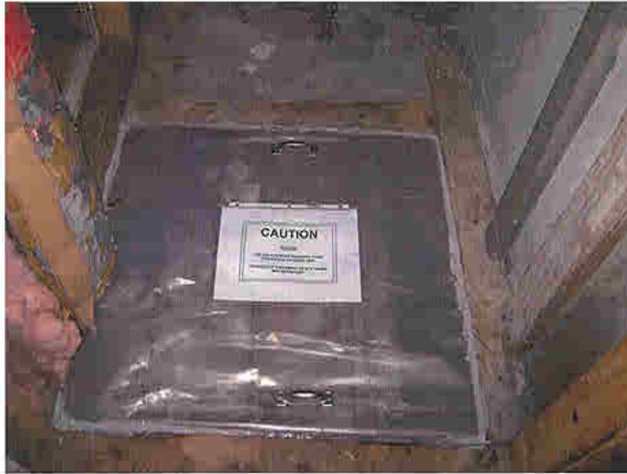
Photo 7: Home #2 sump after being sealed.
