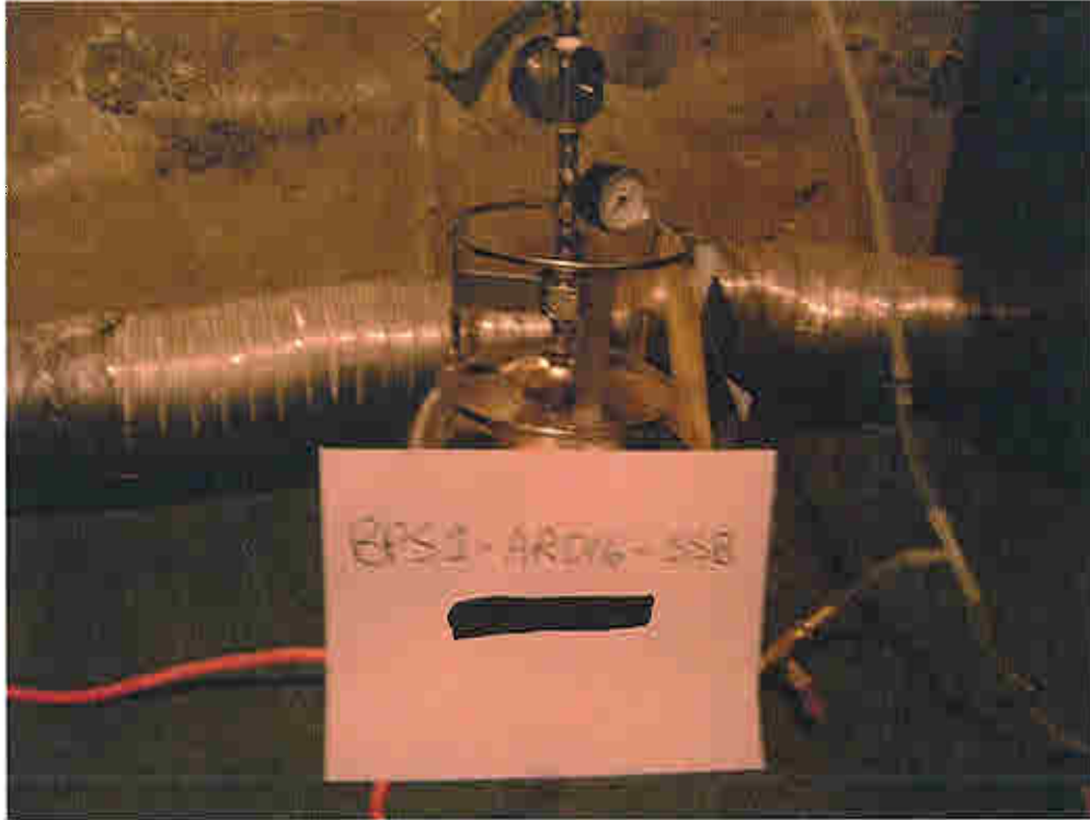
Photo 55: Sub-slab sample location at Home #16.
