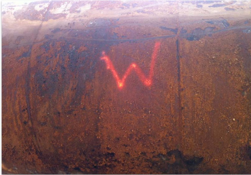
West side of Tank #2
