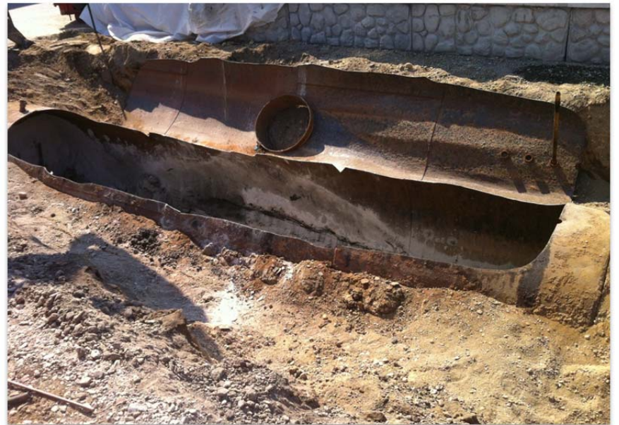
Tank #1 Cleaned of Fluid and Sediment
