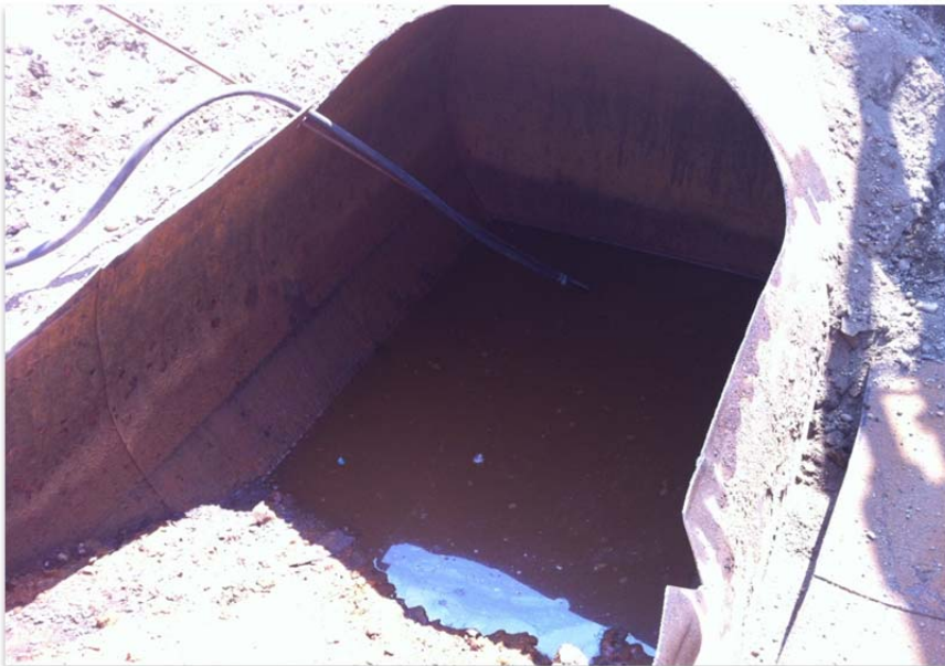
Pumping of Contaminated Water
