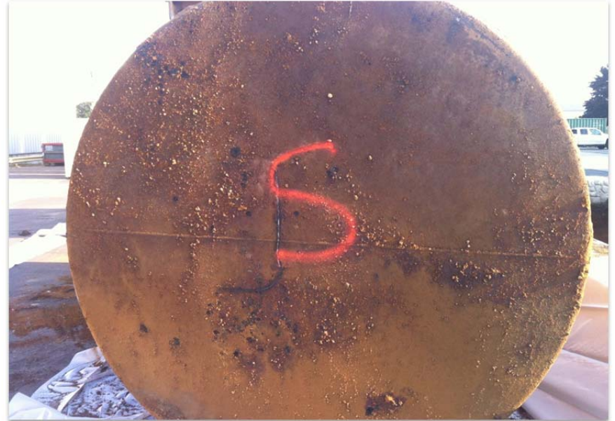
South side of Tank #1
