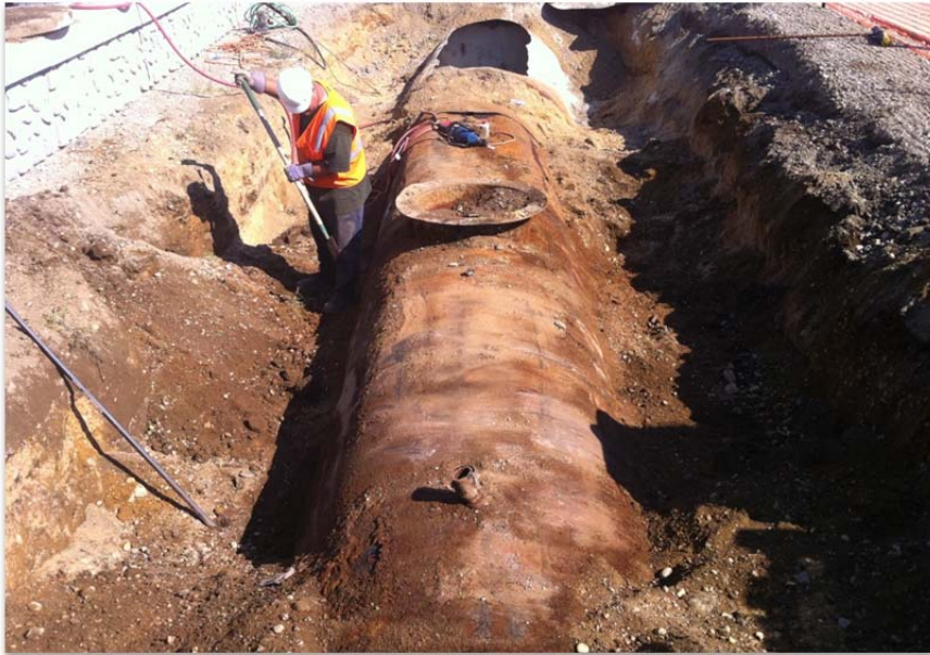
Overview of both Exposed Tanks
