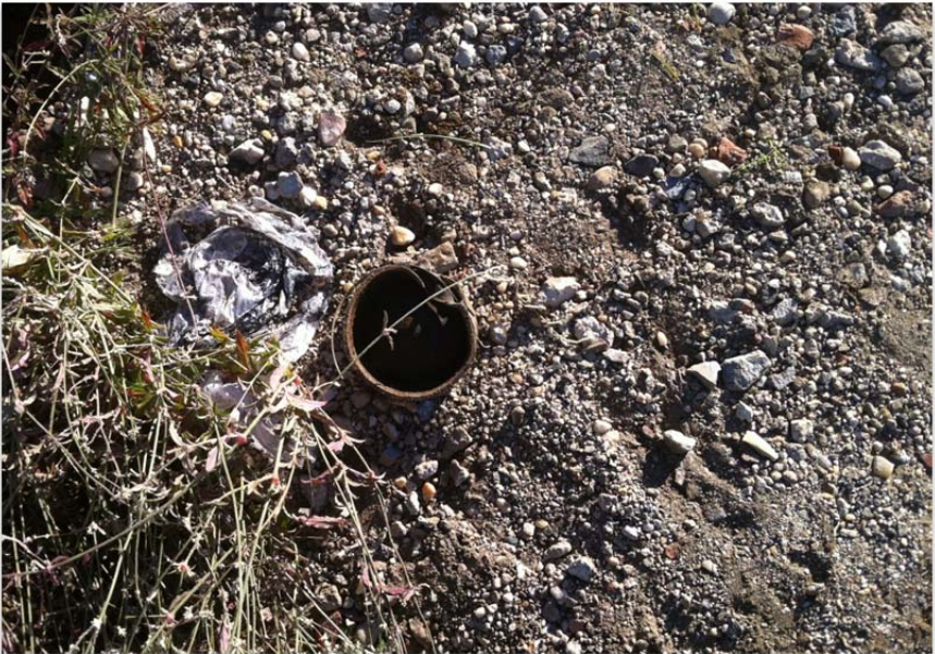
Tank Vent Pipe
