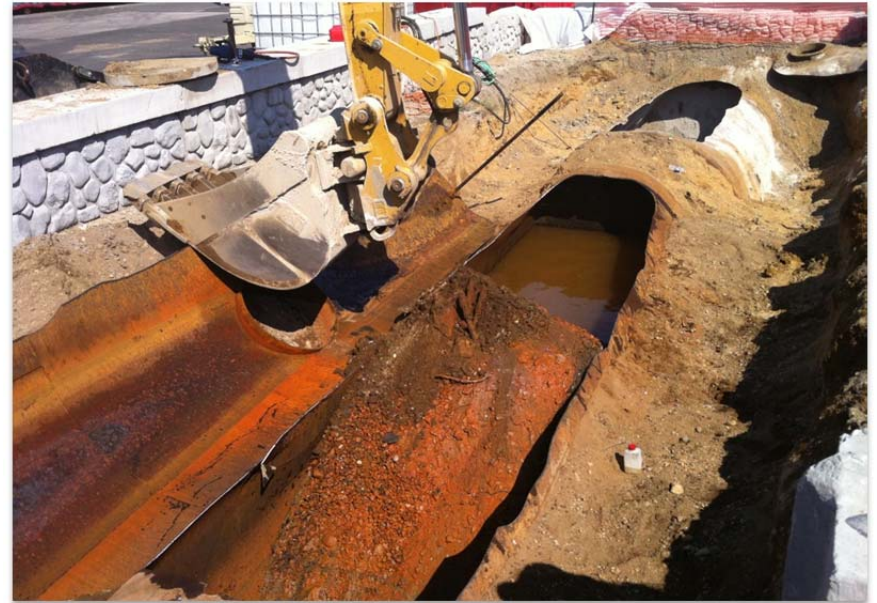
Removal of Tank To Access Fluid and Sediment
