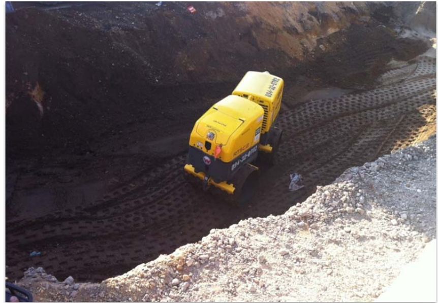
Compaction of Tank Excavation Area
