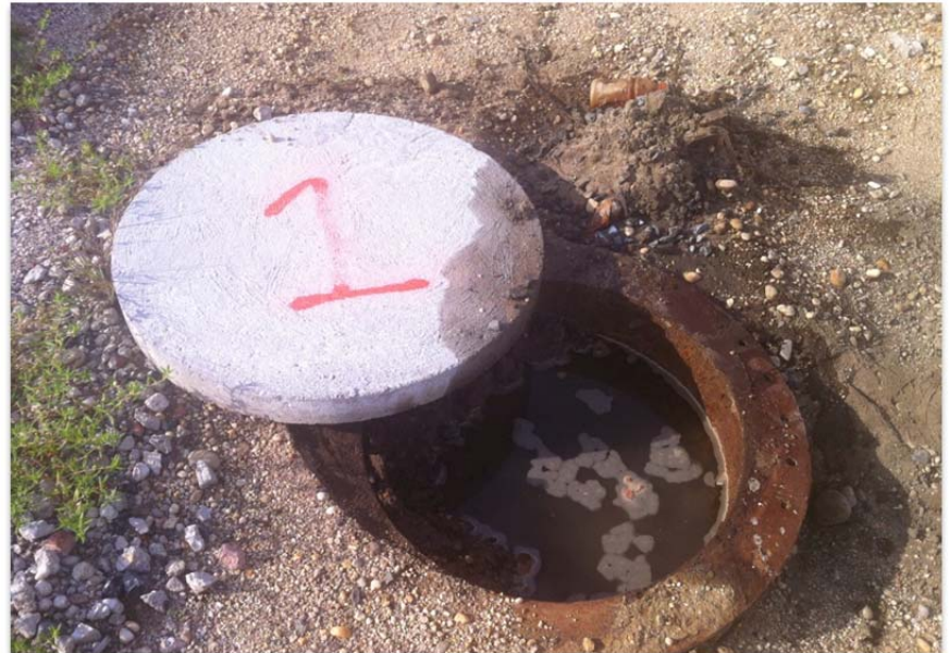
Manway opening Tank 1 South
