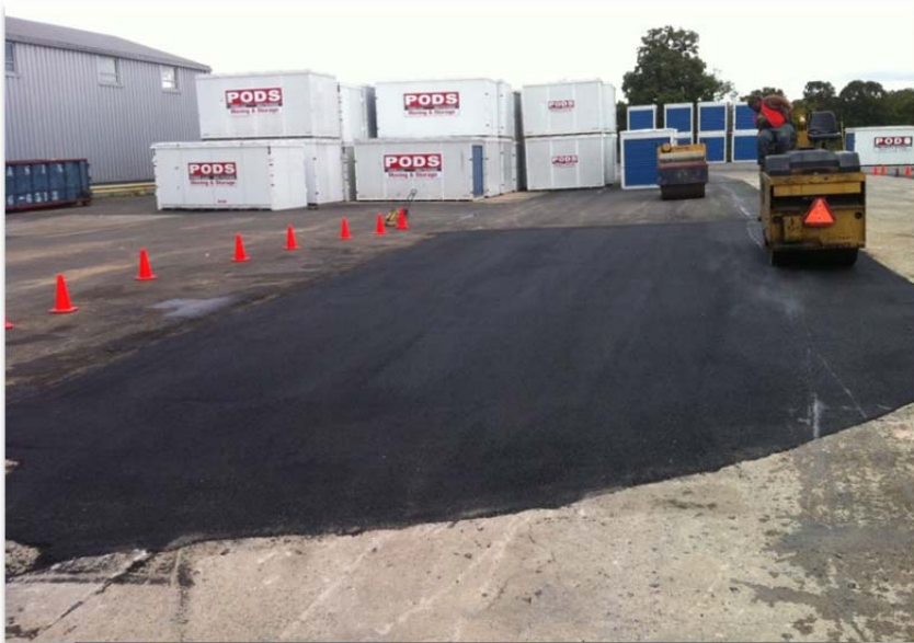
Paving of Excavation Area
