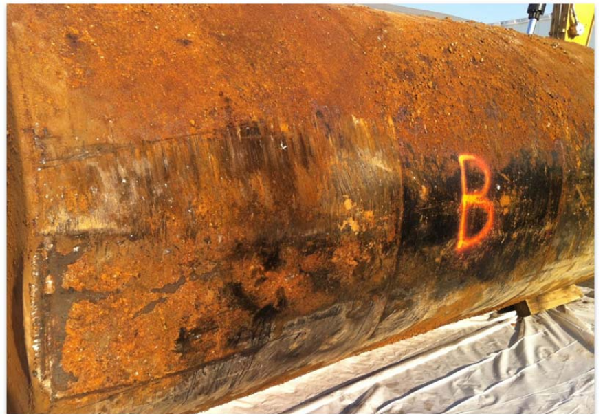
Bottom of Tank #1
