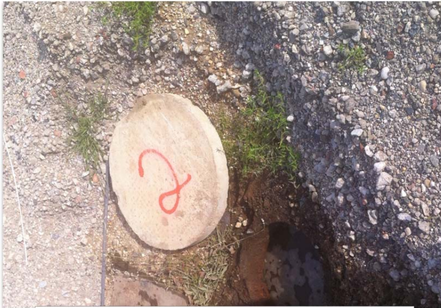
Manway opening Tank 2 North
