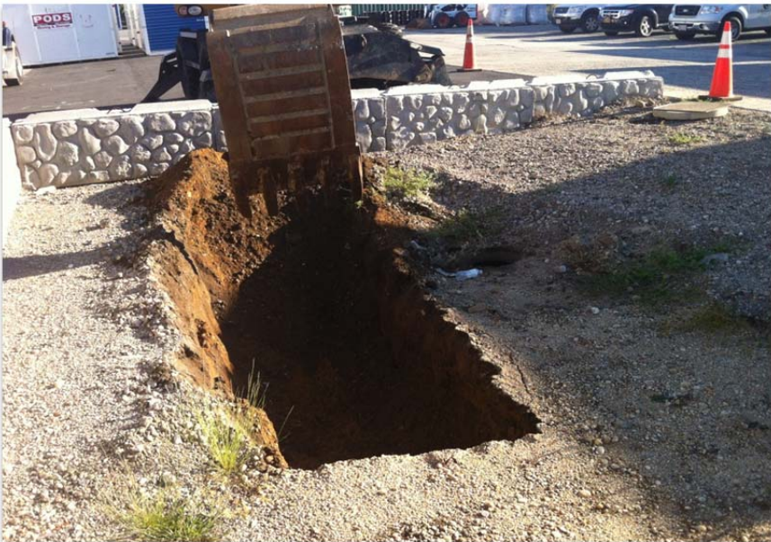
Removal of Overburden
