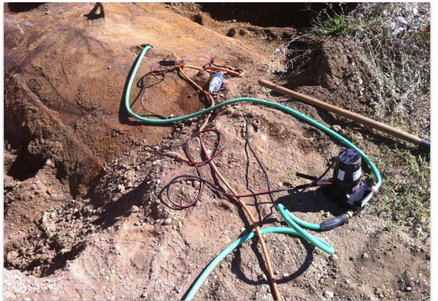
Pump set-up for Fluid Removal
