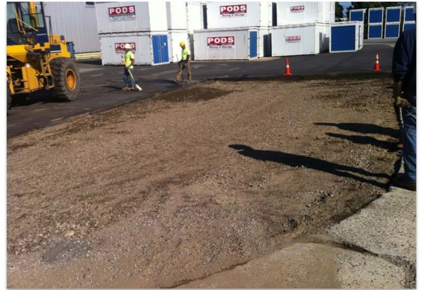
Backfilled to Elevation Acceptable to Facility Manager
