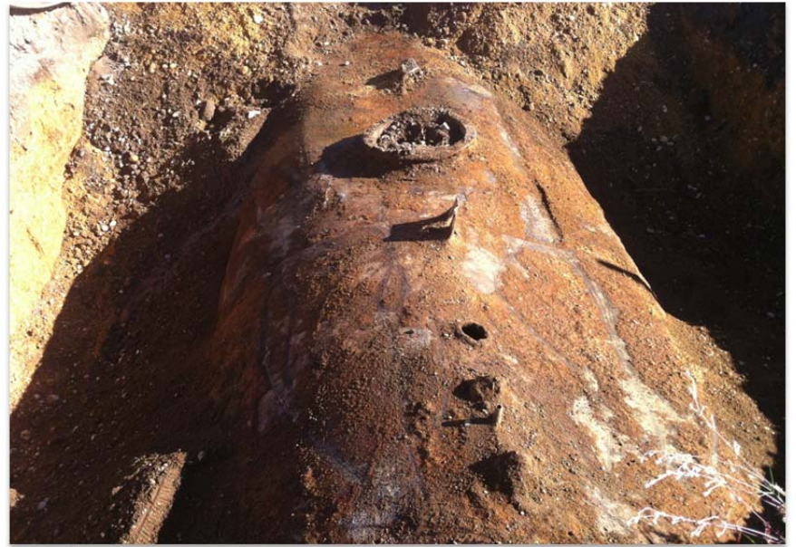
#2 Tank Ready for opening
