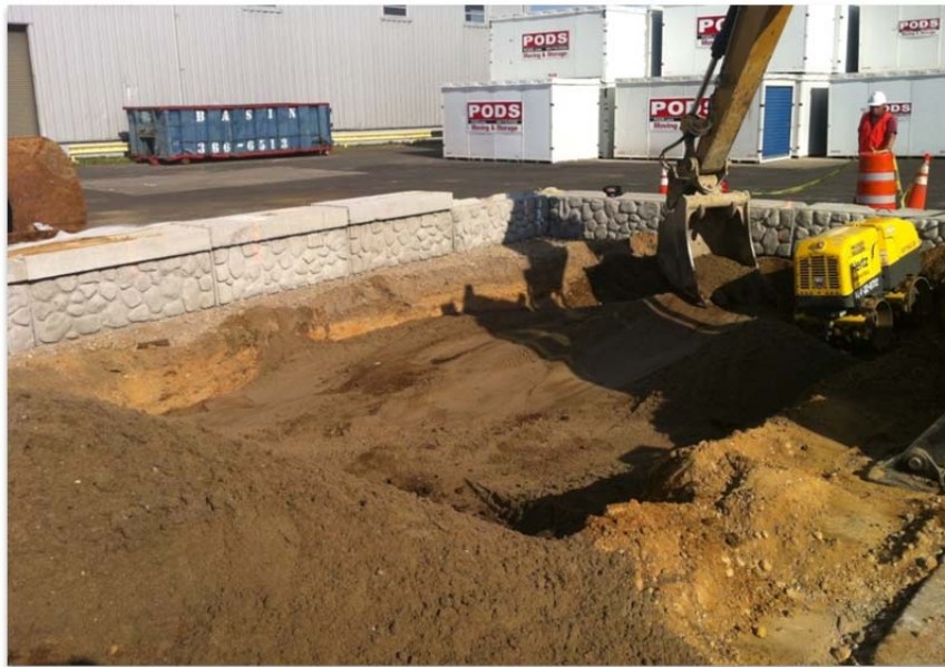
Back-fill Operation of Tank Excavation
