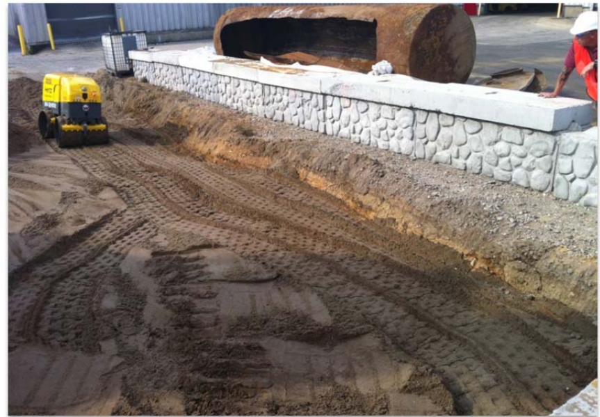
Compaction of Tank Excavation Area
