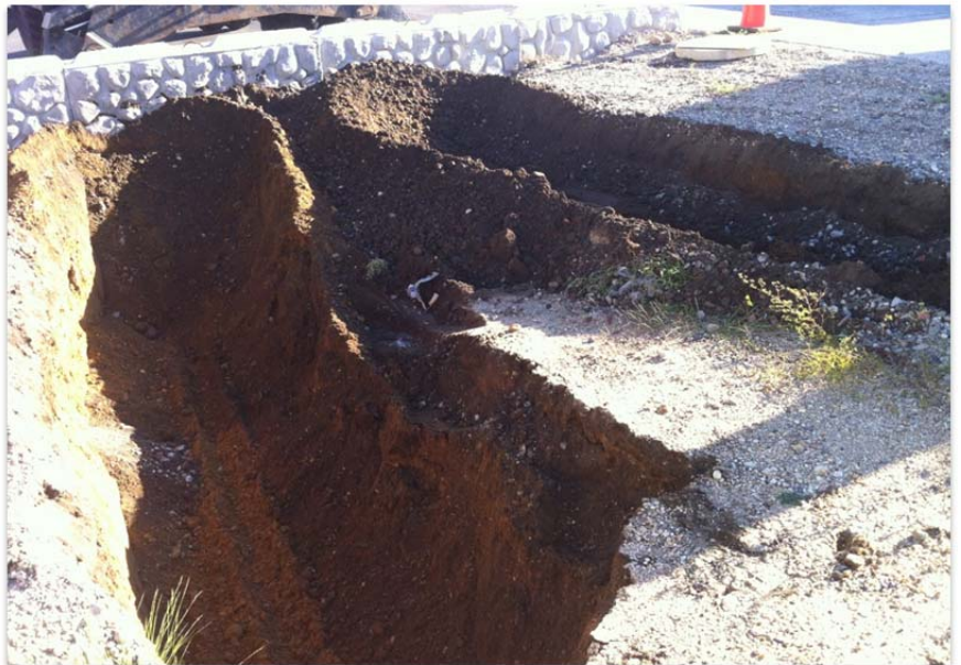
Exposure of #2 Tank
