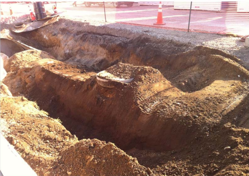
Exposure of Tank #1
