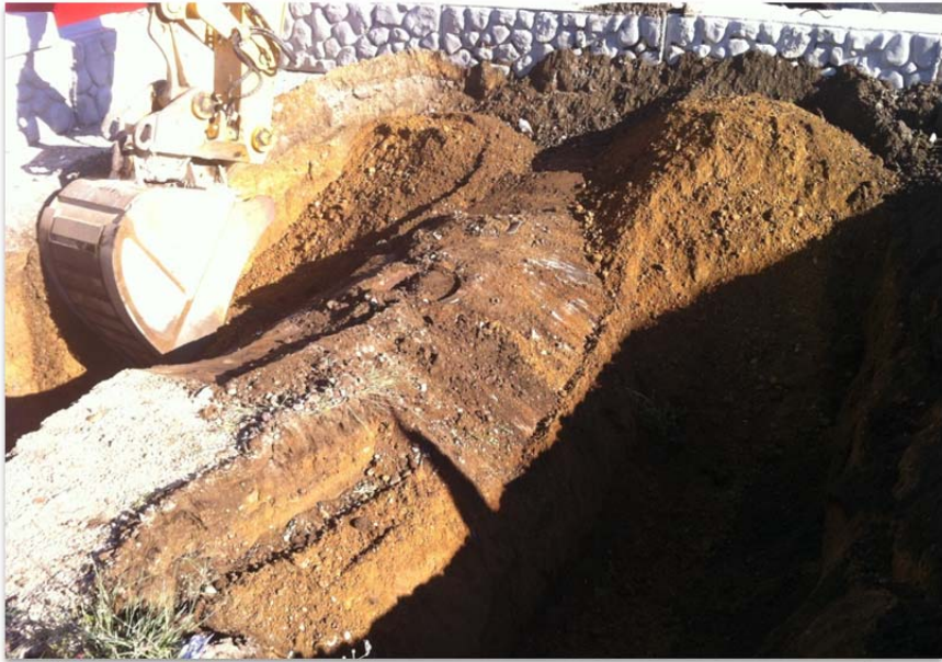
Overburden and Exposure for #2 Tank
