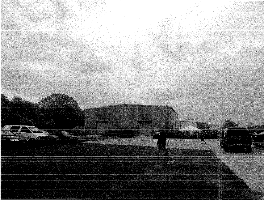
Asphalt cover on Site 3 looking east
