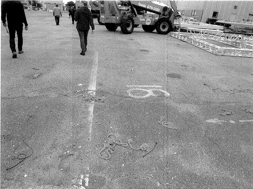
Asphalt cover – Site 3
