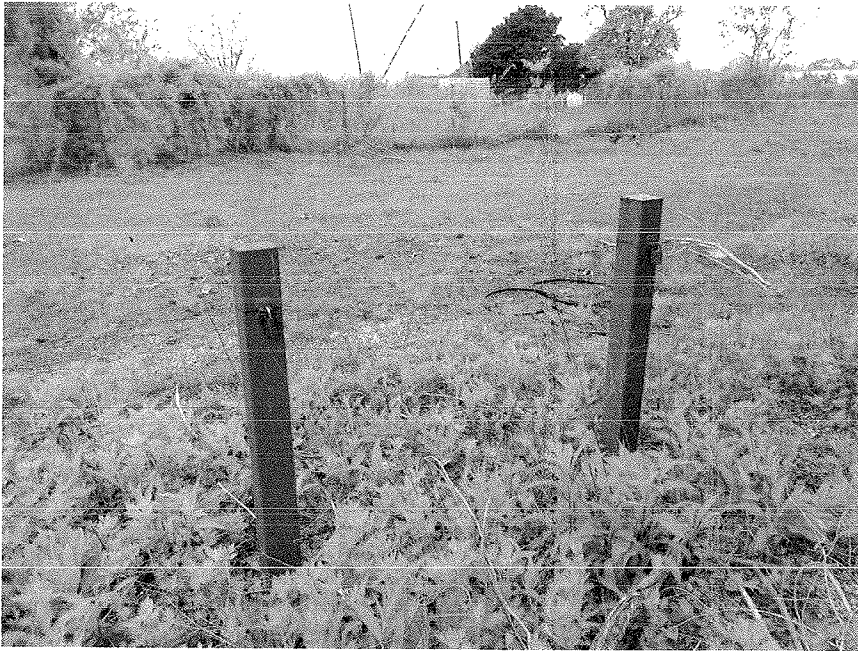
SVE extraction wells 106I&D – Site 1
