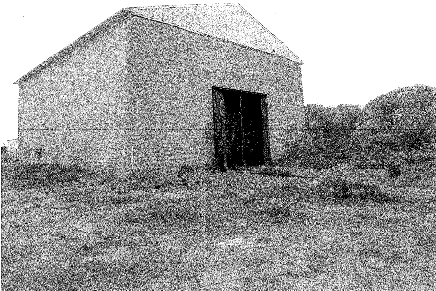
Salt shed - western portion of Site 2
