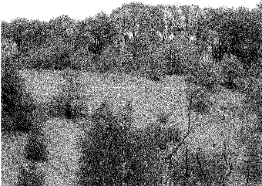
Southern Basin erosion east side – Site 2
