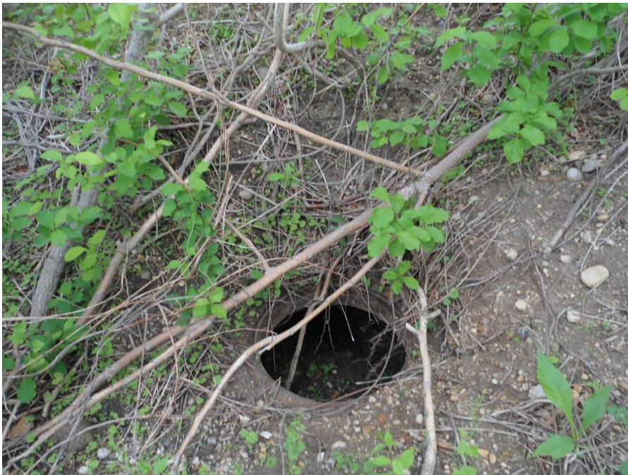
Cess Pool between BPSI-HN- MW27I and BPSI-HN-MW27S – Site 1
