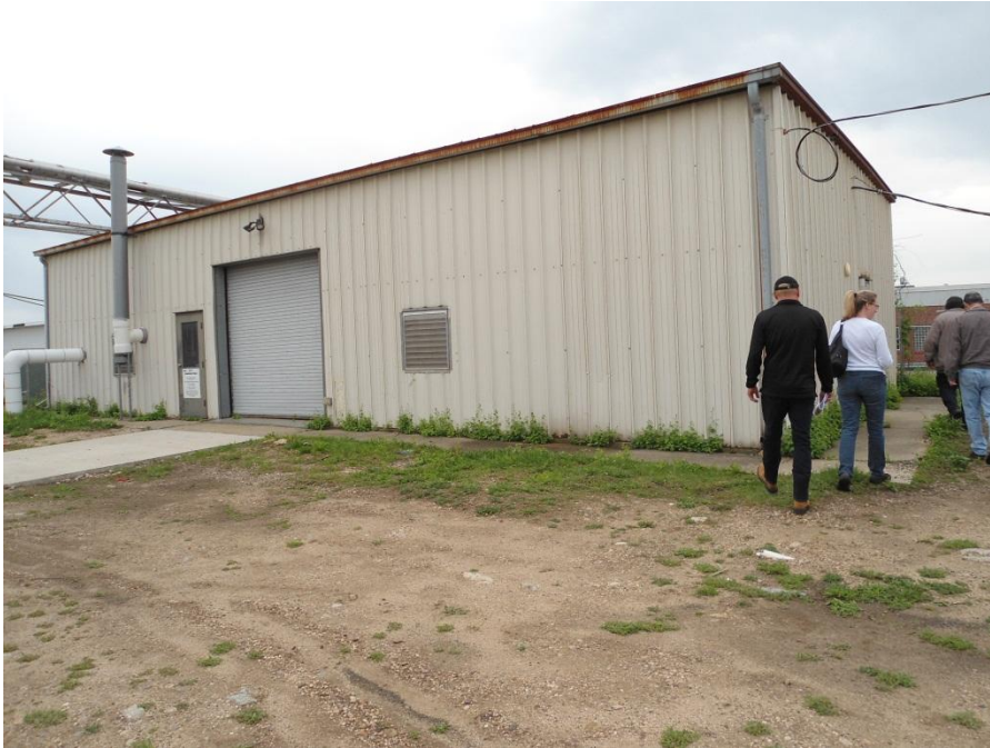
Outside Soil Vapor Extraction System Building (Site 1) - Building located on Site 4
