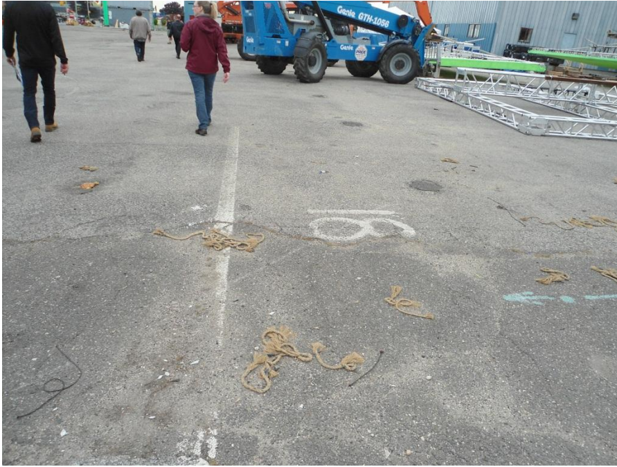
Asphalt cover – Site 3
