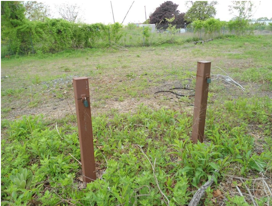
SVE extraction wells 106I&D – Site 1
