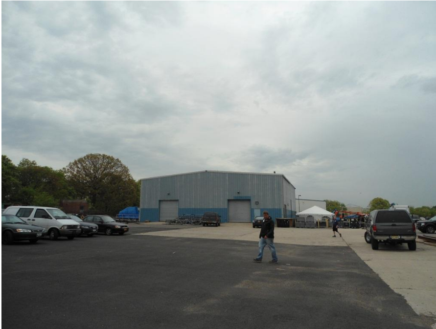
Asphalt cover on Site 3 looking east
