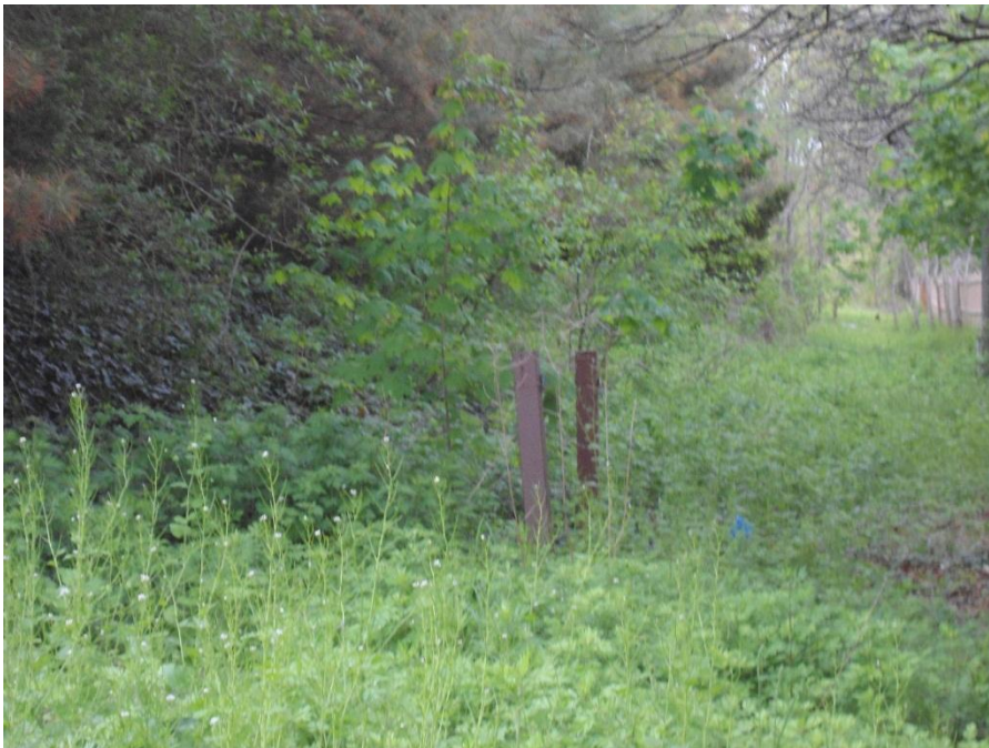
Soil vapor extraction wells – Site 1
