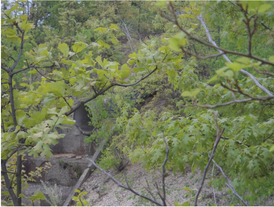
South outfall Southern Basin – Site 2
