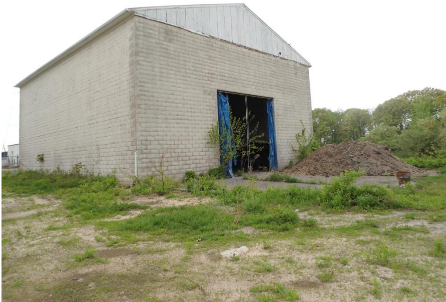
Salt shed - western portion of Site 2
