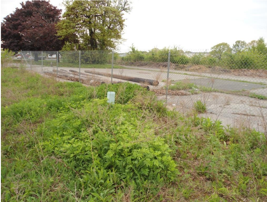
Northern perimeter fence looking northwest – Site 1
