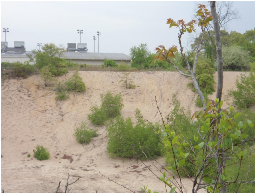
Erosion east side of Southern Basin – Site 2
