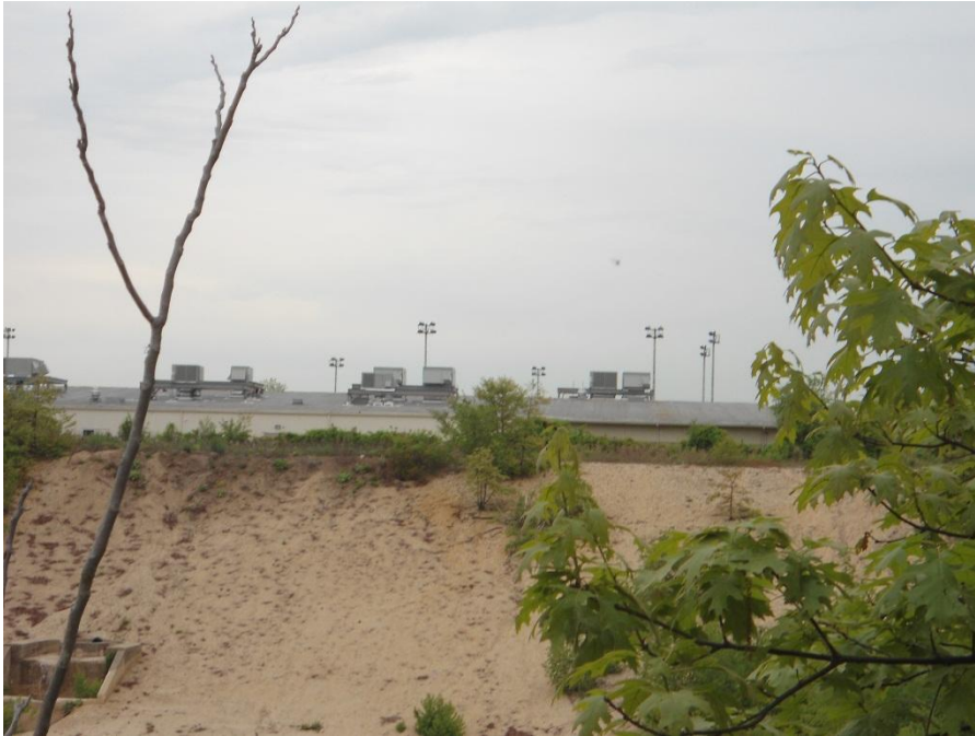
South recharge basin building looking east – Site 2
