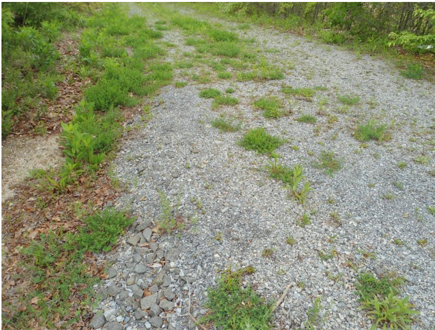
Road cover between east and west recharge basins – Site 2
