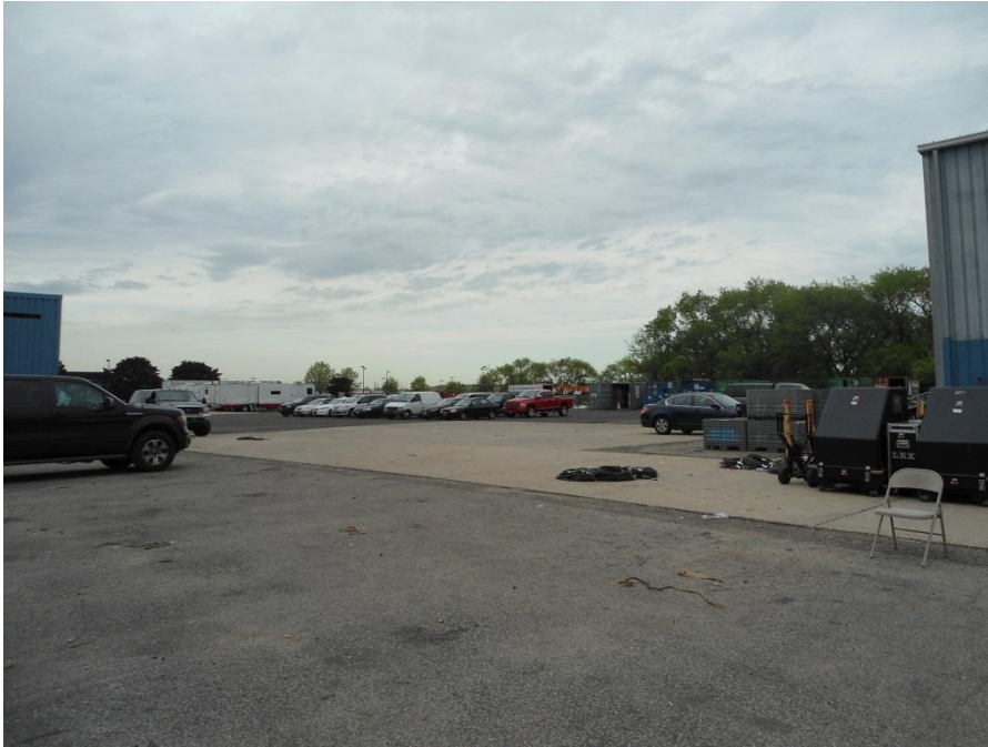
Asphalt that was replaced for movie set – Site 3
