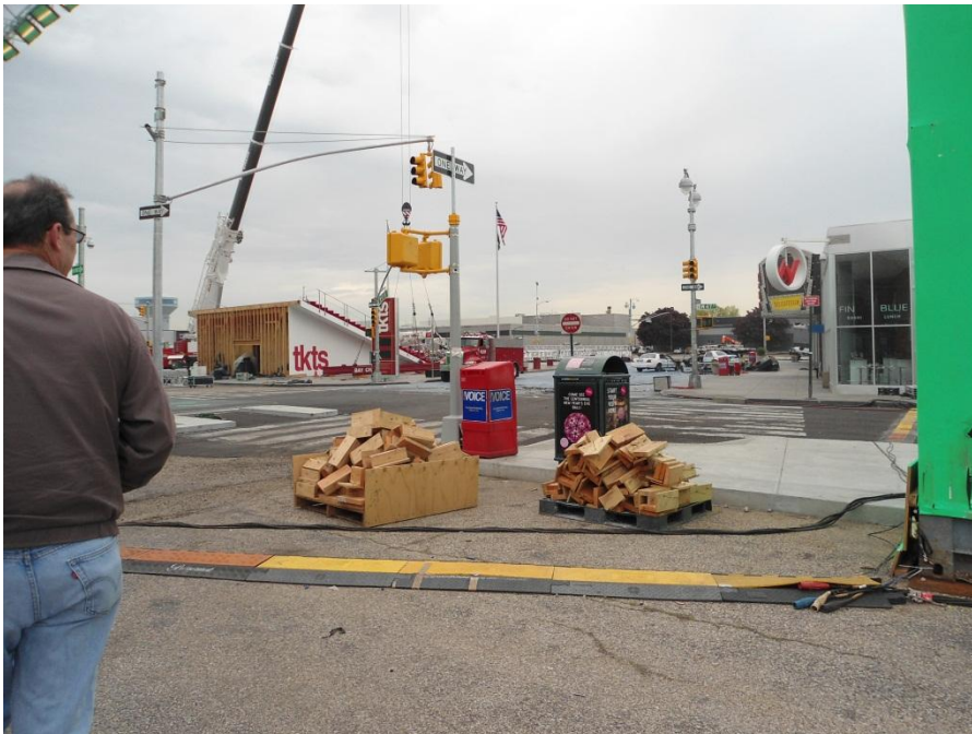
Asphalt cover over Movie Set – Site 3
