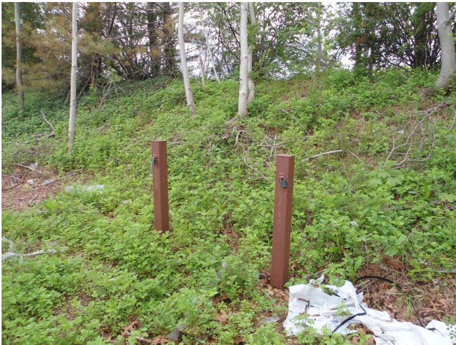
SVE extraction wells 105 I&D – Site 1
