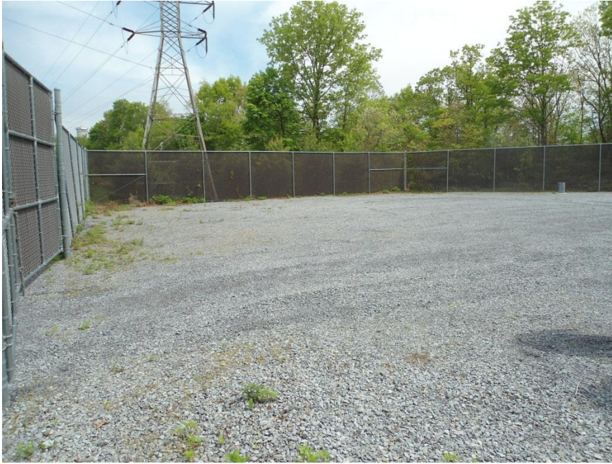
Perimeter fencing - GM38 treatment system – OU2
