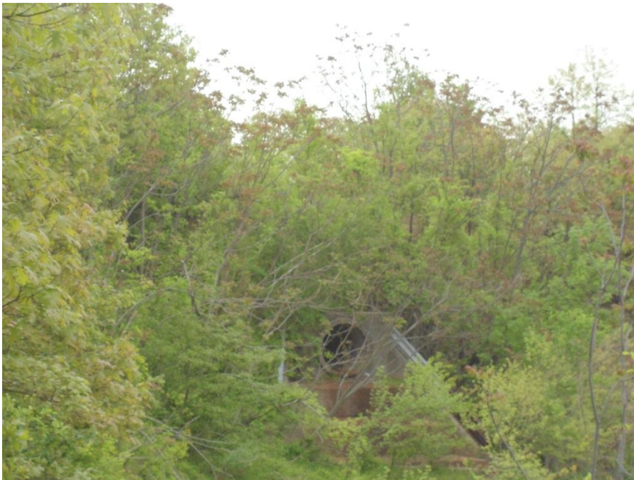
Outfall in Southern Basin – Site 2
