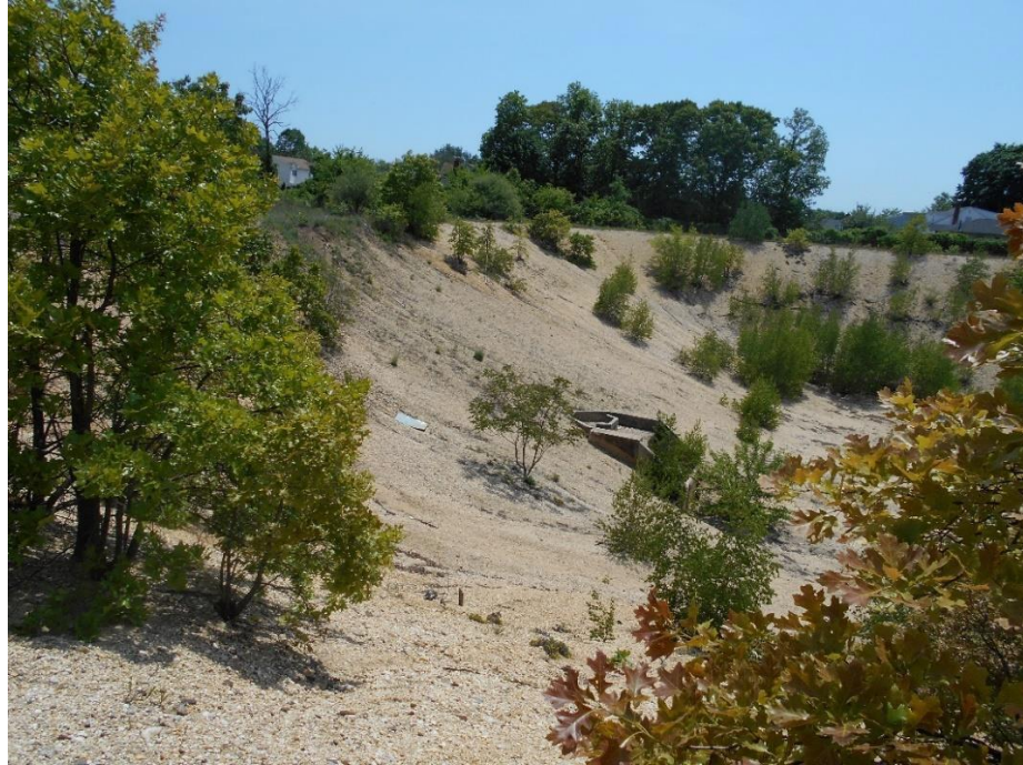
Photo 27: Site 2- Southeast basin facing east, slope erosion
