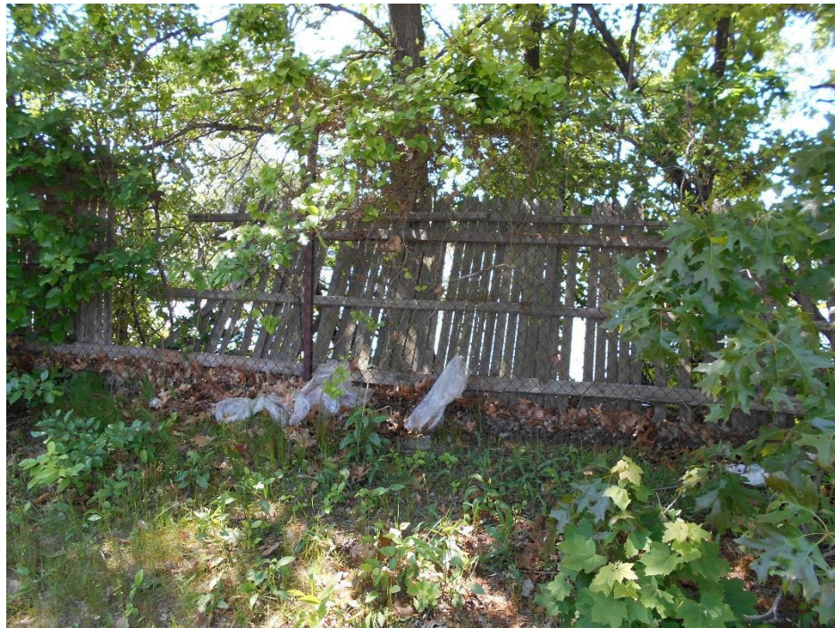
Photo 6: Site 1- Wood fence outside broken
