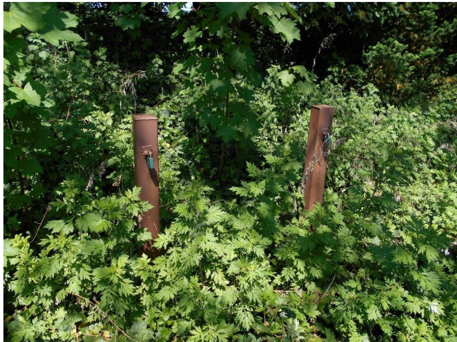
Photo 12: Site 1- SVE 103I + SVE 103D
