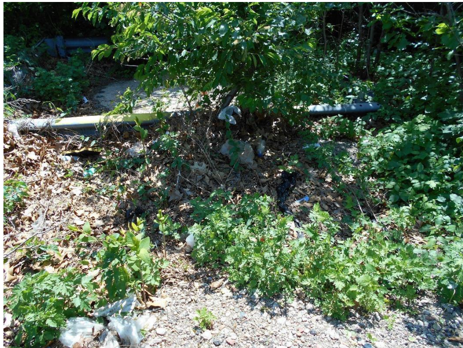
Photo 8 Site 1- Debris at sump
