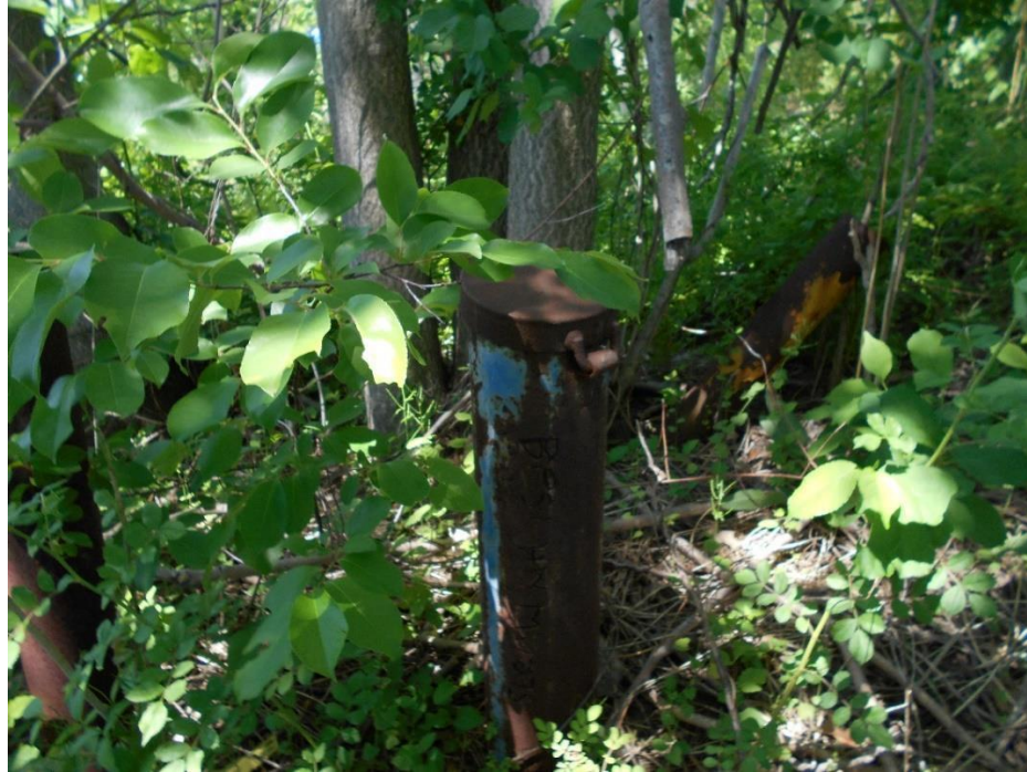
Photo 23: Site 1- BPS1-HN-MW27S, locked on inside, not outside
