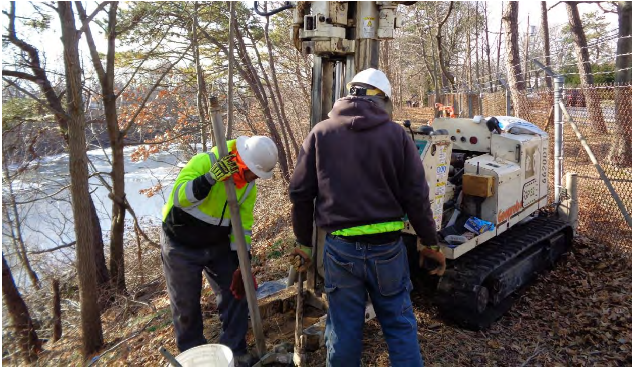
Photo 3: 01/19/2018. Top of north bank, looking west. Soil boring BP-GM38Basin-SB02.
