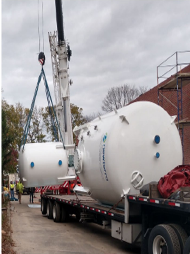
Liquid Granular Activated Carbon Units 1 and 2.
