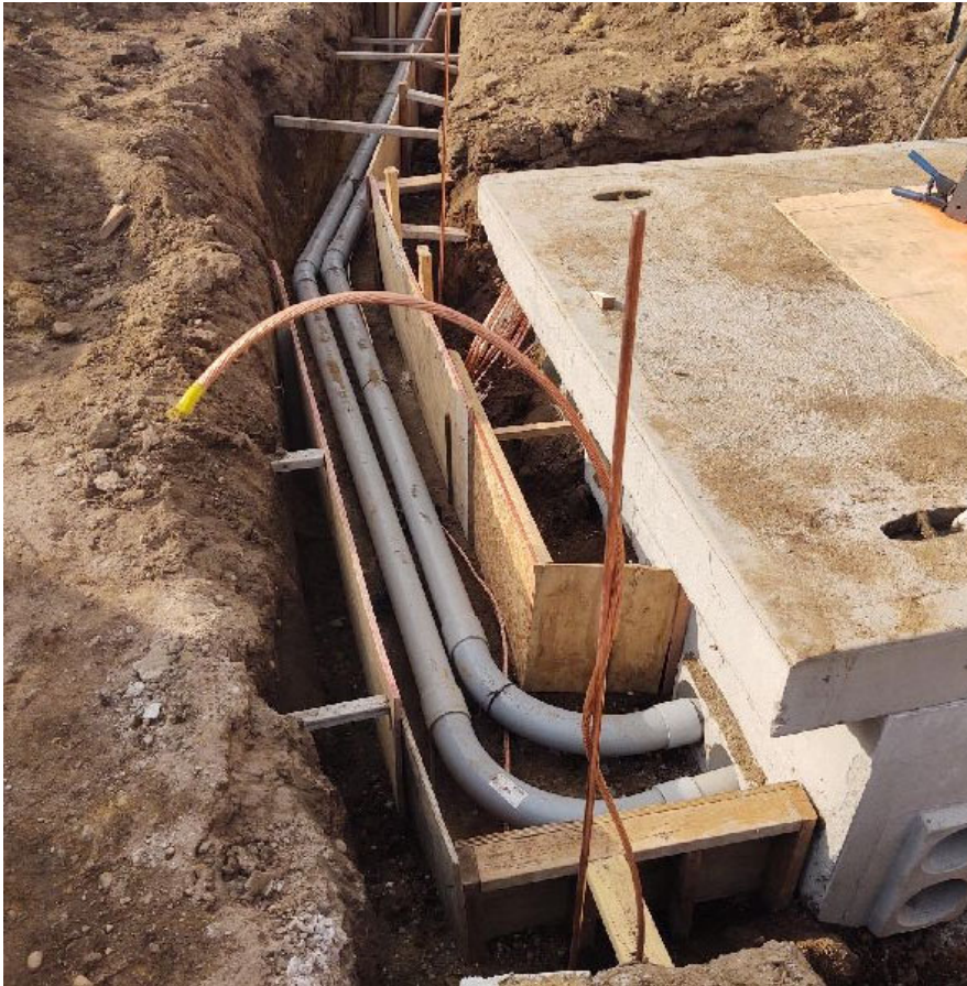
March 2023. GWTP concrete electrical duct bank formwork
