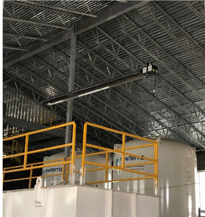
April 2023. Radiant heaters and FRP installation
