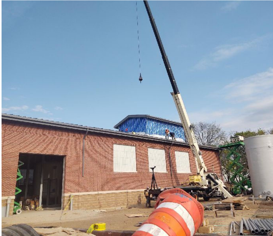
April 2023. Metal roof panel installation. Looking northwest.
