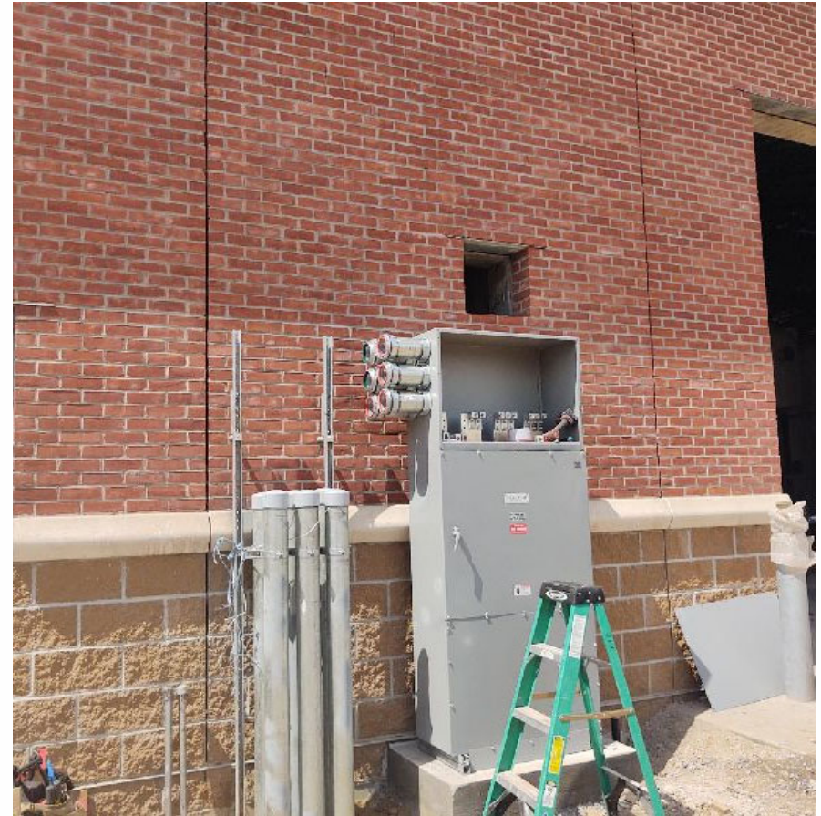
April 2023. GWTP electrical box and stub ups installed
