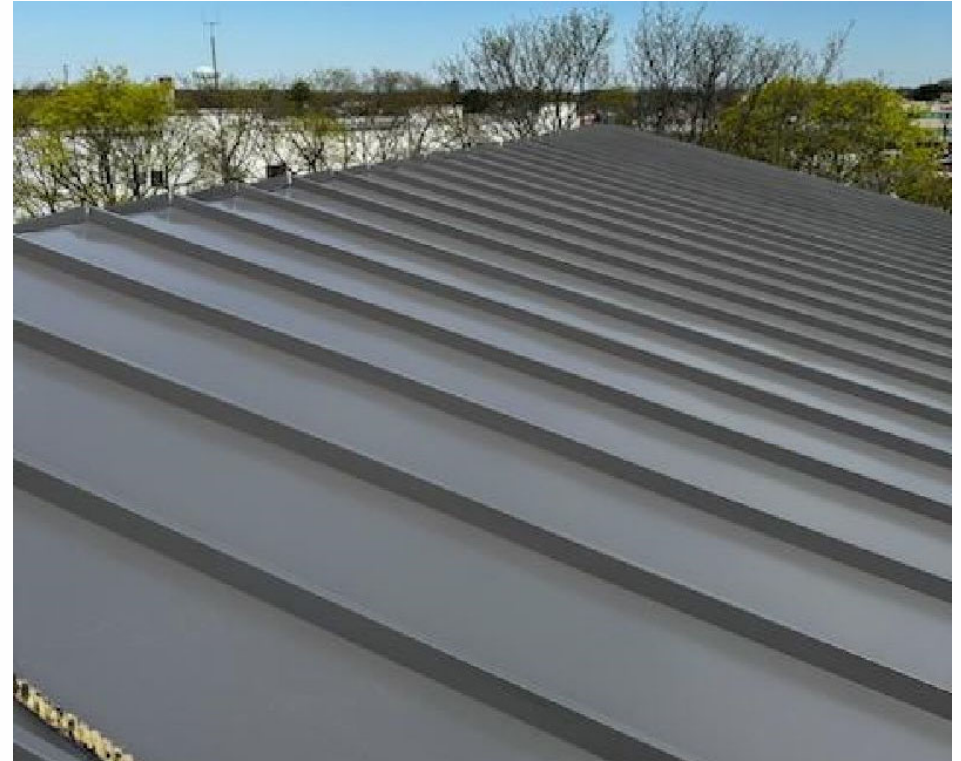
April 2023. Roof panel installation, elevated AST tower.
