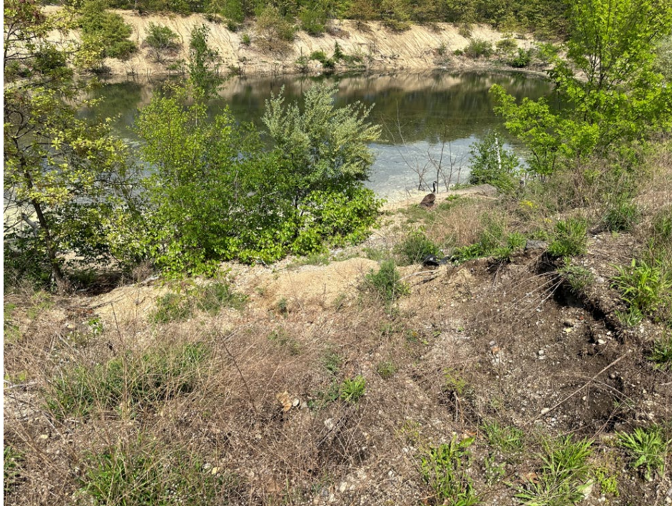
View looking north of northeast settling pond with erosion on southwest corner
