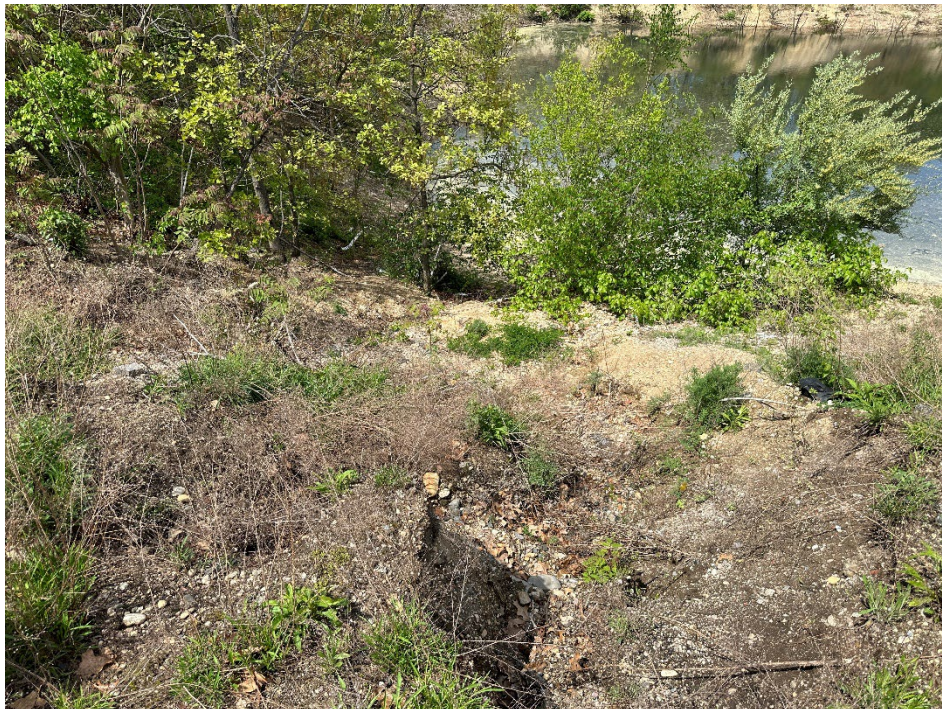
View looking north of northeast settling pond with erosion on southwest corner
