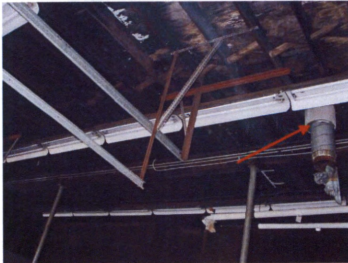
3. 03-13 - Remove the flue pipe and transite insulator pipe.
