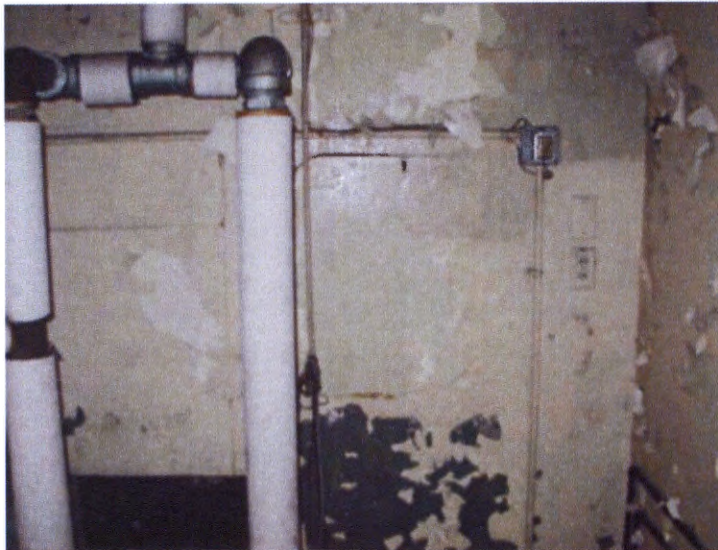
2. 03-13 - Remove transite wall and ceiling panels
