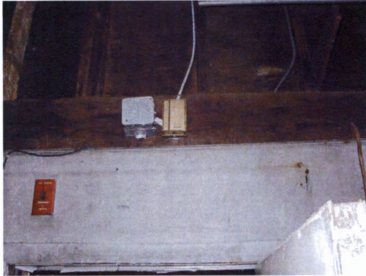
5. 03-13 - Remove and recycle mercury thermostats
