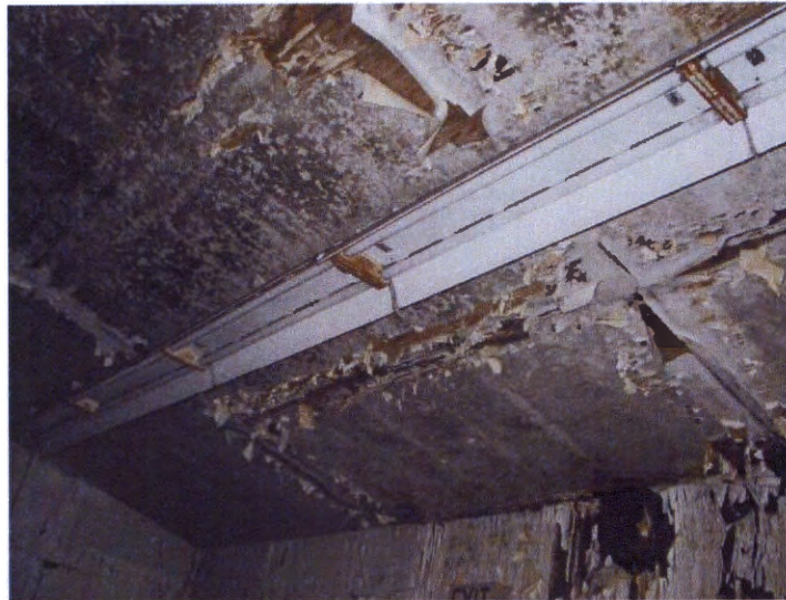
4. 03-13 - Remove fluorescent lamps and PCB lamp ballasts
