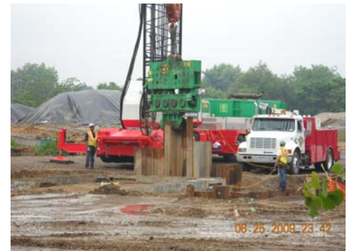
Sheet Pile Driving with Crane
