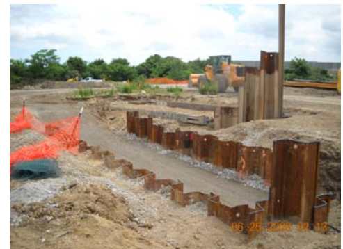
Compaction of excavation area 2
