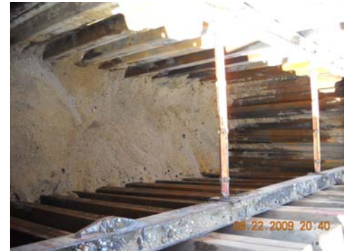
Completed excavation area 2
