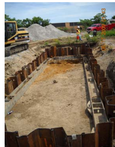
Completed Sheet Piling Around Area 2
