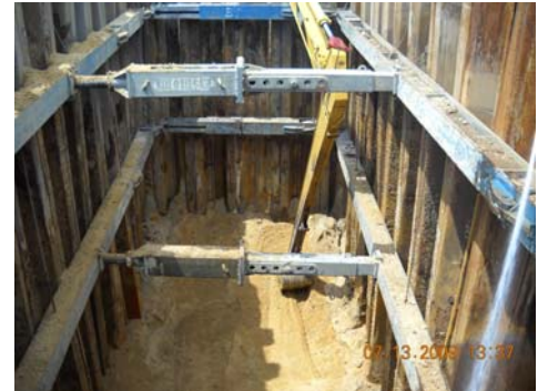
Excavation of Area 3
