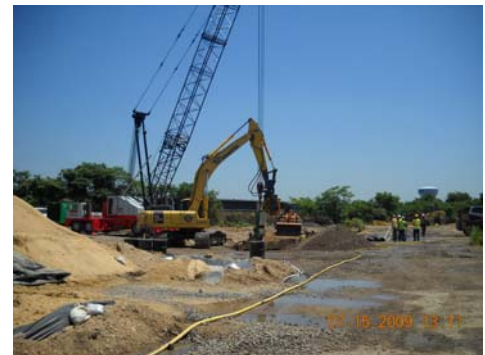
Removal of Sheet Piles from Area 3
