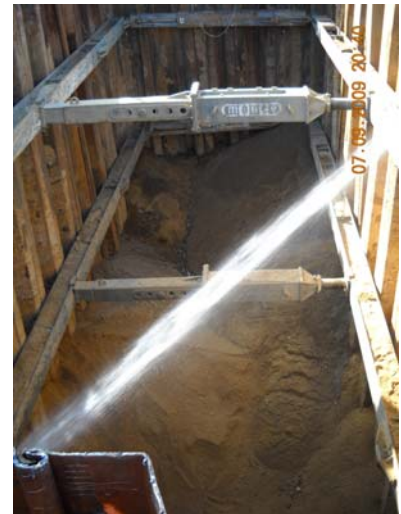
Excavation of Area 3
