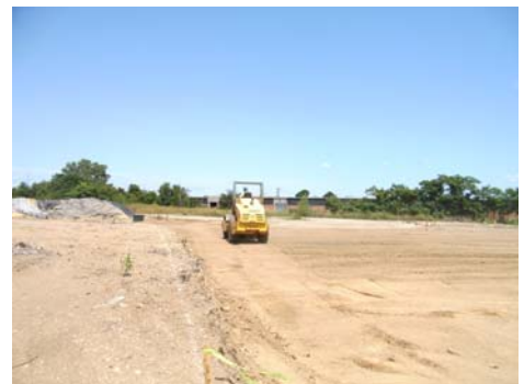
Compacting Scraped Soils Area
