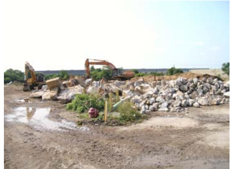
Consolidating concrete for disposal
