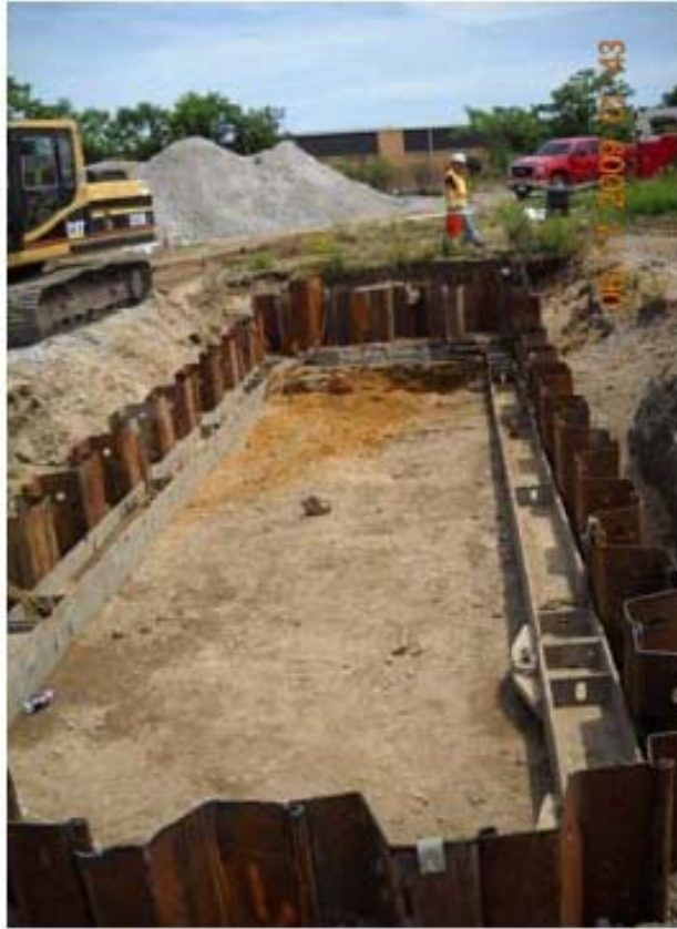
Completed Sheet piling Around Area 2
