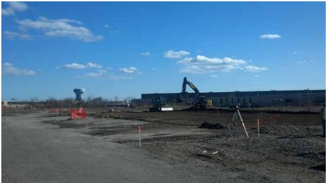
Construction of Material Staging/Containment Area
