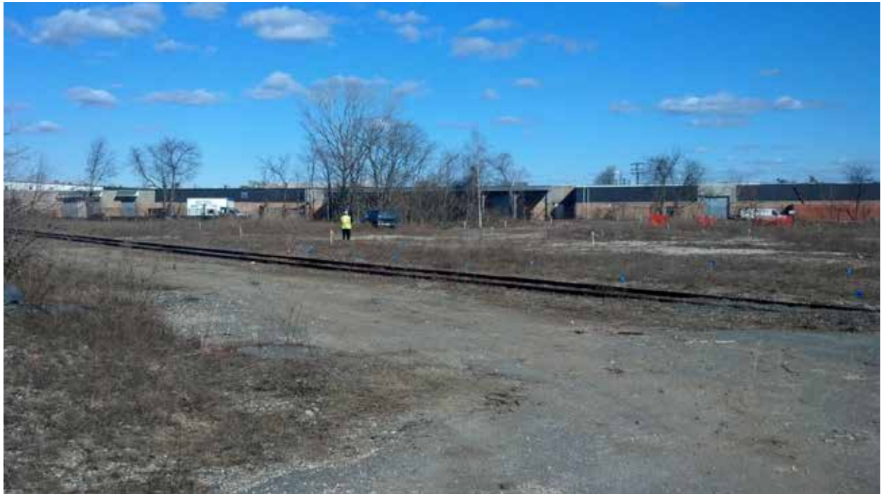
Surveying & Marking Proposed Excavation Limits
