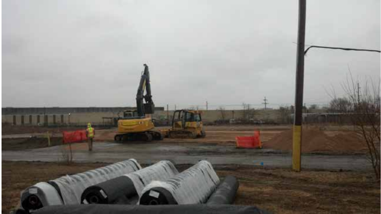
Construction of Material Staging/Containment Area
