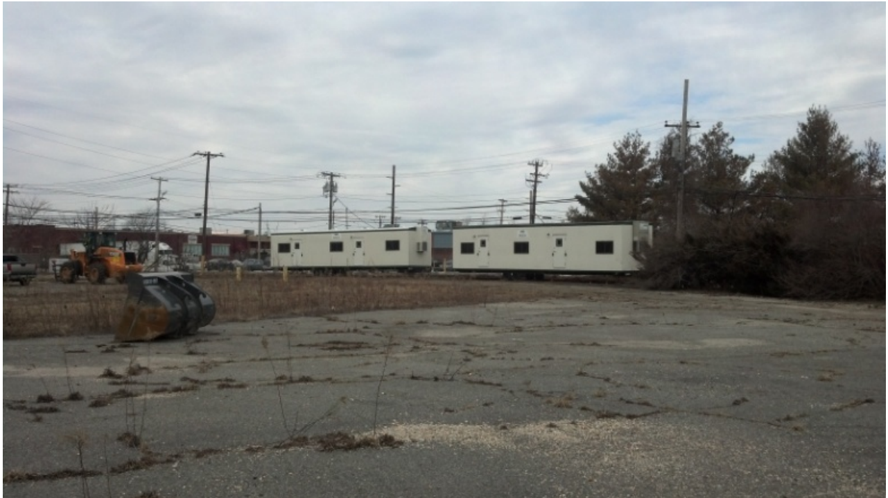
Mobilization of Field Office Trailers
