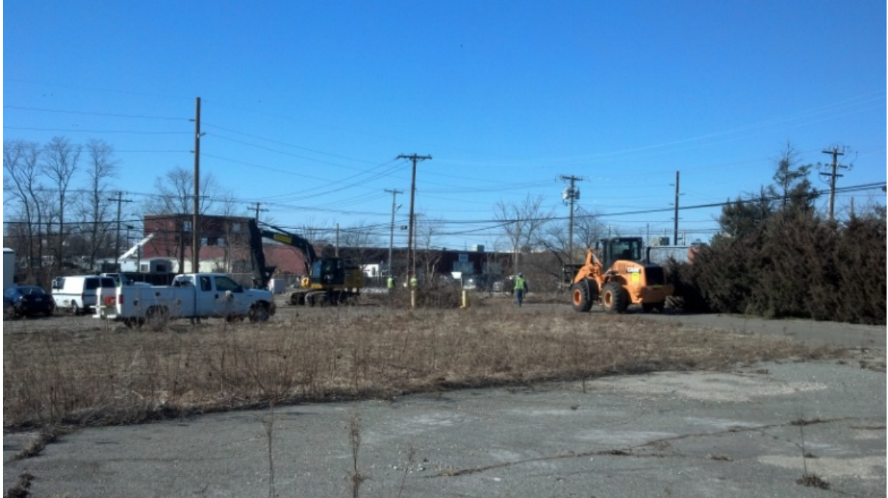
Mobilization of Equipment
