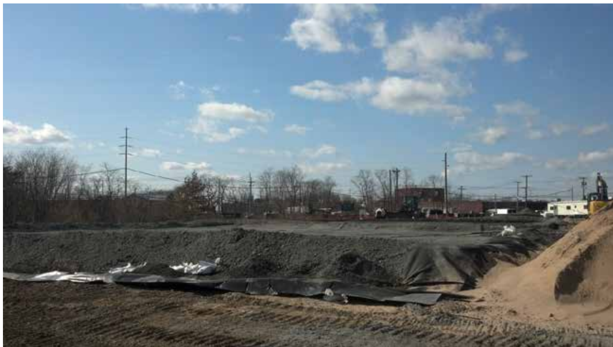
Construction of the Material Staging/Containment Area
