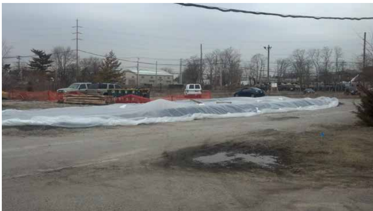
Construction of the Decontamination Pad (6 Mil Poly Cover Visible in Photo is Intended to Reduce Rain Water Accumulation)
