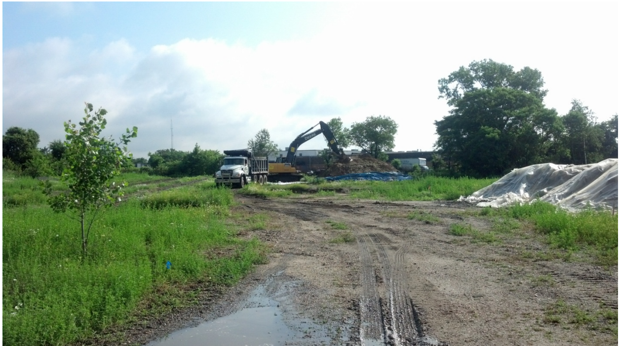
Loading of Tri-Axle Trucks with SP-1 Soil for Offsite Non Hazardous Soil Disposal
