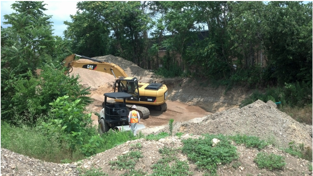
Compaction of Backfill of Area 20A
