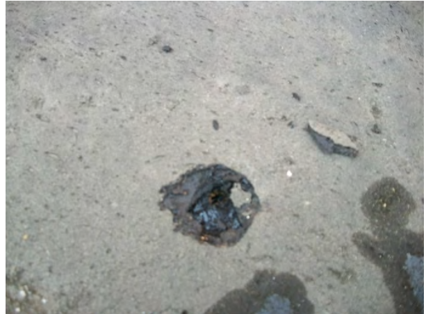
HA-32: Built-Up Roofing associated with North Entry Roof
