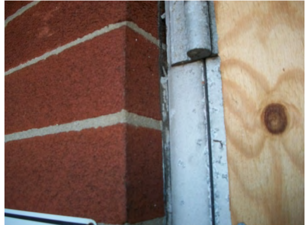
HA-25: White Exterior Door Caulking
