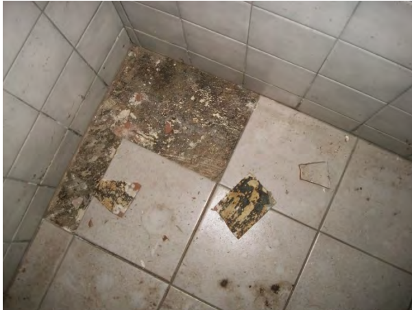
HA-11: Grout associated with 6" Gray Ceramic Floor Tile; HA-12: Gray and Black Adhesive associated with 6" Ceramic Floor Tile
