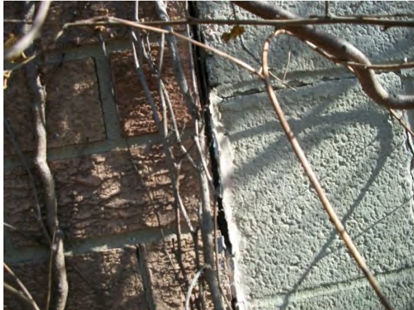
HA-24: White Expansion Joint Caulking
