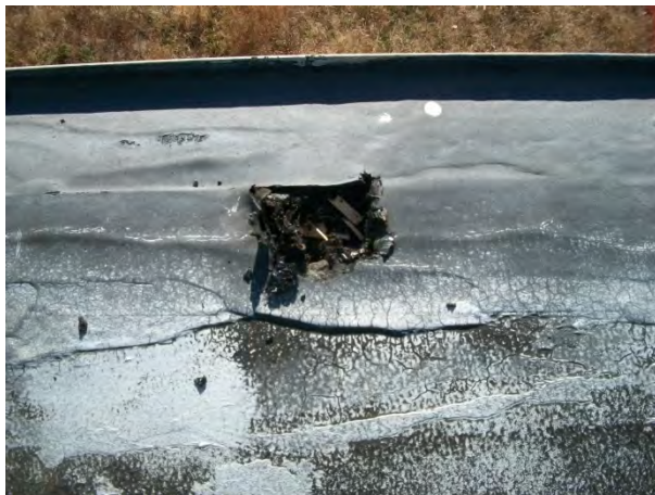
HA-29: Built-Up Roofing associated with Perimeter and Penetrations
