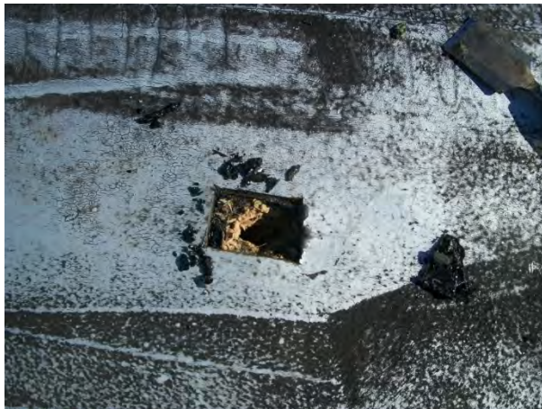
HA-26: Silver Coated Rolled Asphalt Roofing; HA-27: Built-Up Roofing associated with Main Roof Field
