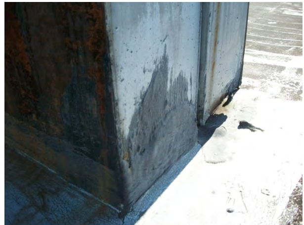
HA-28: Flashing Cement associated with Perimeter and Penetrations
